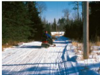
This is a common example of a comfortable clearance zone adjacent to a groomed and tracked trail. The clearance zone is especially important where trees and brush are present on downhills. Note that by limiting the clearance zone, trail "creep" can be controlled, as can cross-country travel.
