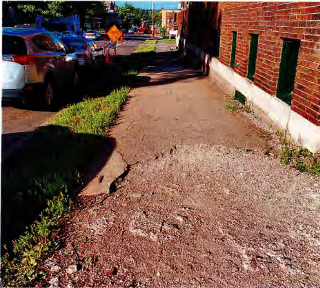
Anticipated sidewalk vault at the 710 E. Second Street.
