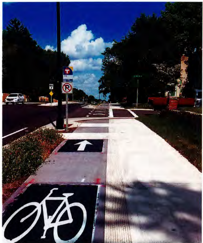
Off-Street Bicycle Accommodation Location: S. Minneapolis, MN – Photo Credit, James Gittemeier, DSMIC
