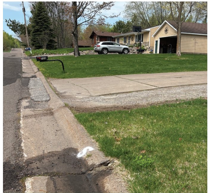
Existing patch at driveway and drainage from sump pump.
