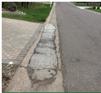
Brick paver driveway with bituminous in the gutter pan.
