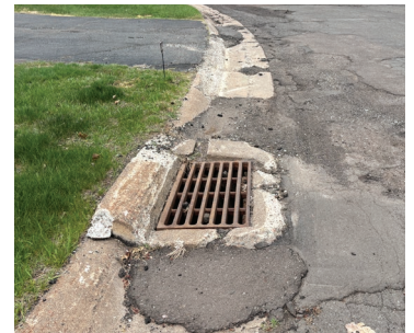
Vaulted catch basin and damaged curb and gutter.
