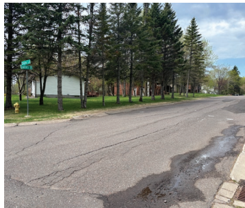
Pipe heave and drainage not in gutter.
