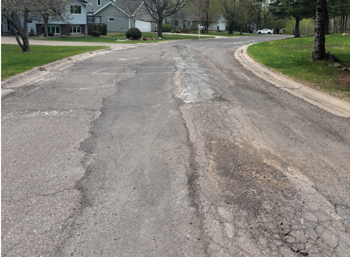
Pavement damage from pipe heave.
