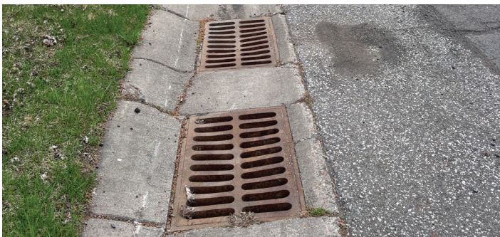
Older style rectangular catch basins in deteriorating S-type curb & gutter.
