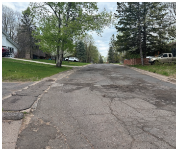
Poor pavement condition and driveway patch.
