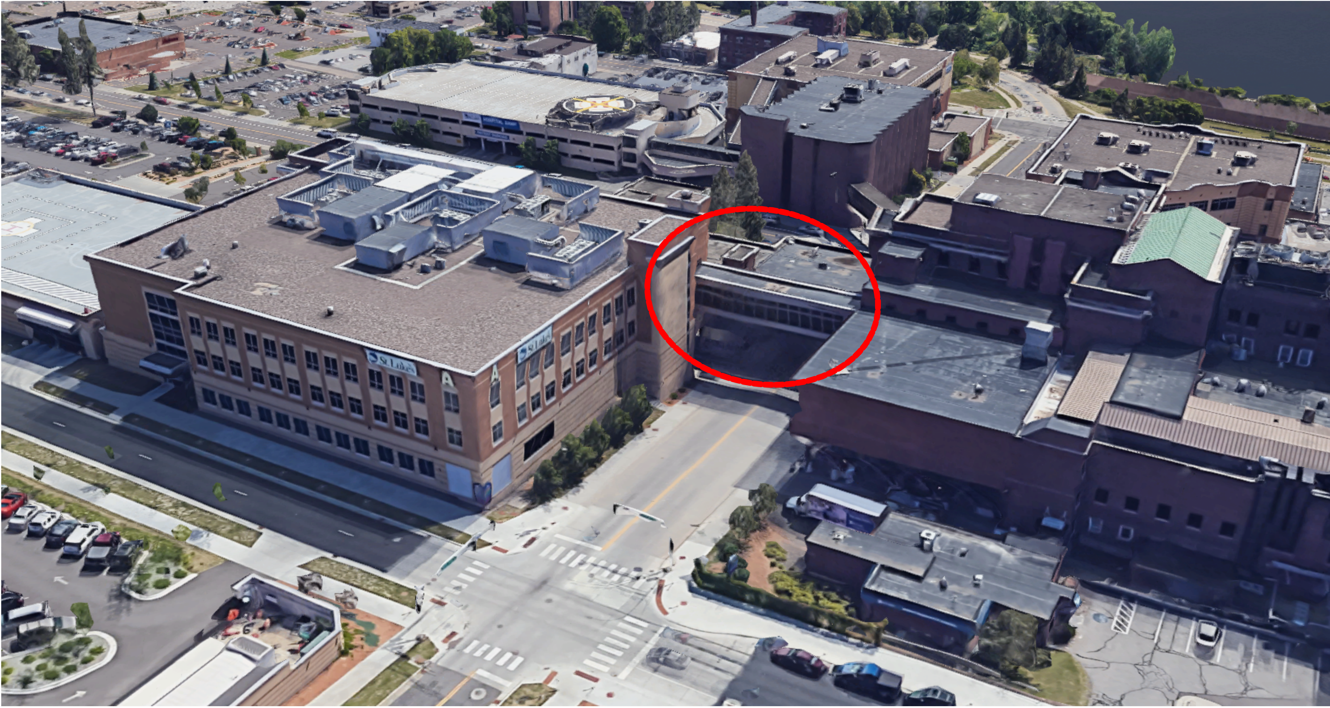
2 SITE CONTEXT - LOOKING EAST SCALE: 12" = 1'-0"
