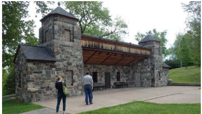
No operational restroom facilities in pavilion building
