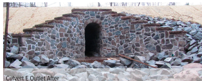
Culvert E Outlet After
