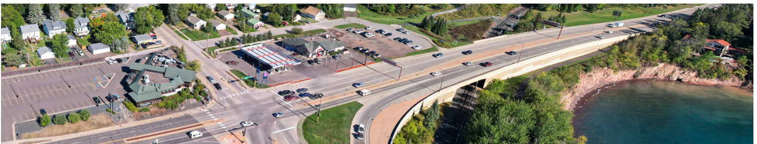
35W and London Road. One of the residences to be inspected is shown on the far right of the image on the shoreline below London Road.
