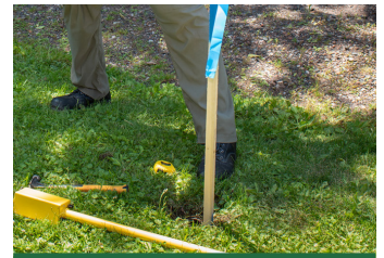
Locating the curb stop.
