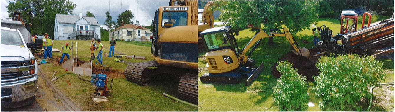
i New water main and service line June 26 th and 27 th , 2017.
