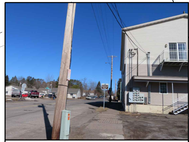
C SITE OVERVIEW [LOOKING NORTHWEST]
