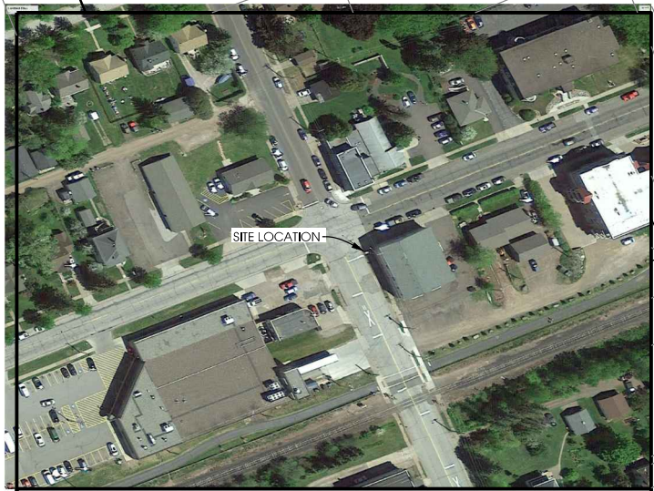
A AERIAL OVERVIEW
