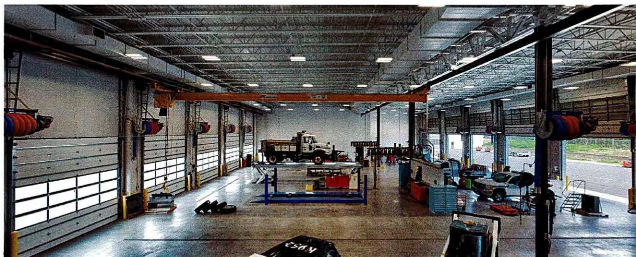
Fleet Maintenance Facility
