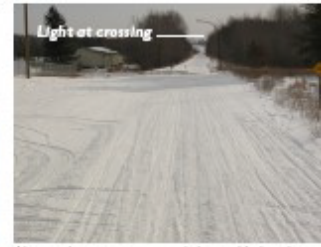
Along with proper signage, a light is added at this trail crossing to improve safety. The flatness and straightness of this rail conversion reduced the visual cues associated with identifying this intersection, warranting the addition of the light.
