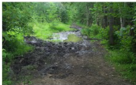
This otherwise sustainable snowmobile corridor is not well suited to summer ATV use, as the photo clearly illustrates. An ongoing occurrence of this type of impact only leads to more restrict uses, sometimes even for those the trail was designed to accommodate.
