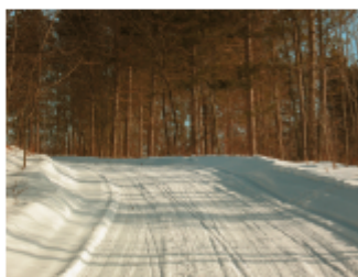
These classic two-way snowmobile trails are groomed to between 12 and 14 feet wide. The trail on the left runs through a northern forest where sightlines are more limited, which helps keep riding speeds lower. In the middle photo, the long abandoned rail-grade trail is very flat with long sightlines. Here, too, 12 to 14 feet is adequate to accommodate two-way traffic.
