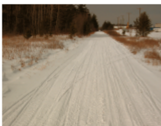
These classic two-way snowmobile trails are groomed to between 12 and 14 feet wide. The trail on the left runs through a northern forest where sightlines are more limited, which helps keep riding speeds lower. In the middle photo, the long abandoned rail-grade trail is very flat with long sightlines. Here, too, 12 to 14 feet is adequate to accommodate two-way traffic.
