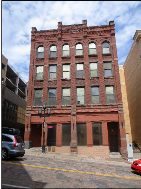
12 Lake Avenue (Historic Name: Tremont Hotel)
