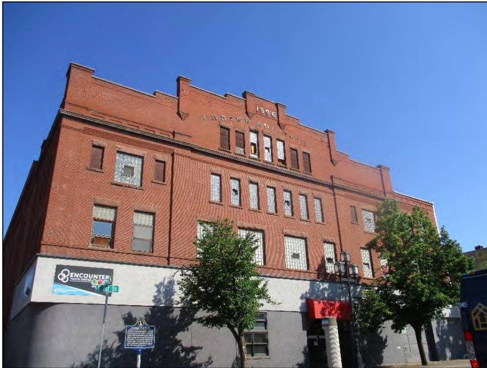
201-207 East 1st Street (Historic Name: Duluth Armory)
