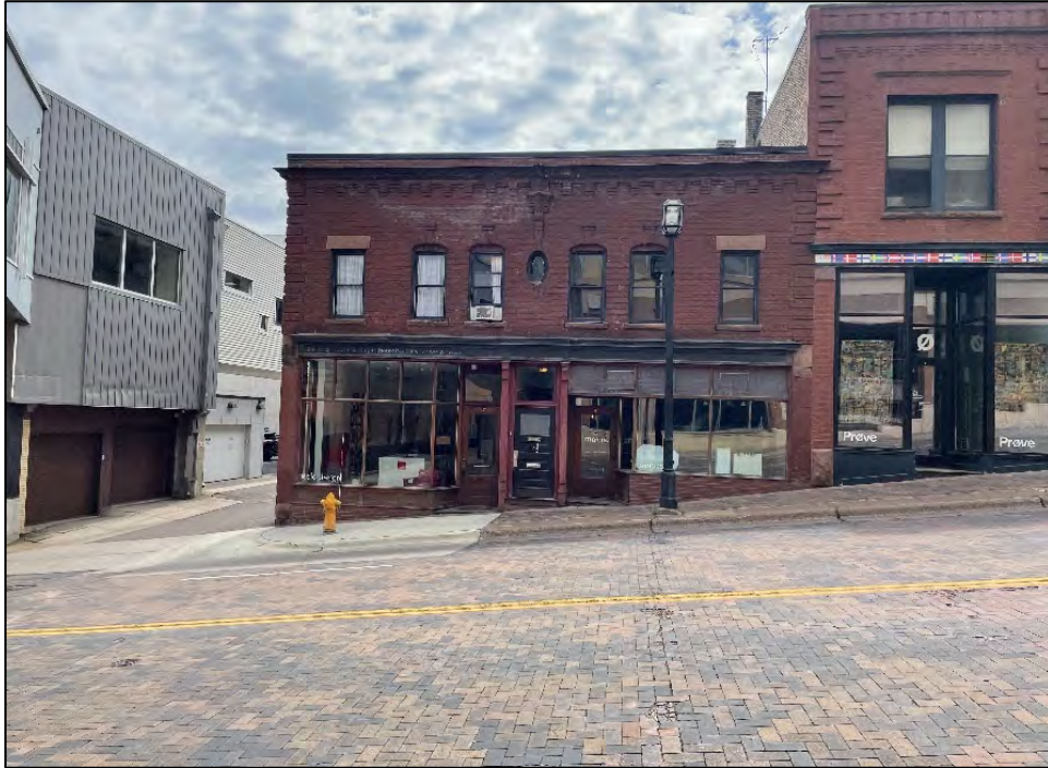
Photograph 15: Storefronts like this example located along Lake Avenue should be maintained.
