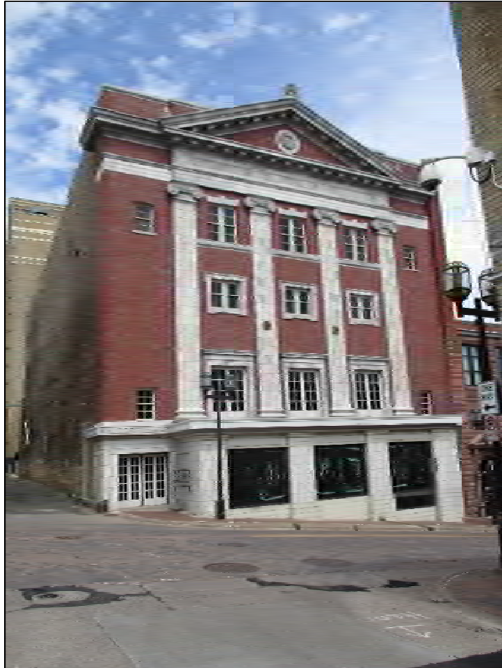
Photograph 5: View of the Classical Revival Orpheum Theatre on N. 2 nd Avenue E. Note the pediment, ionic pilasters, and keystone window lintels at the 3 rd story.
