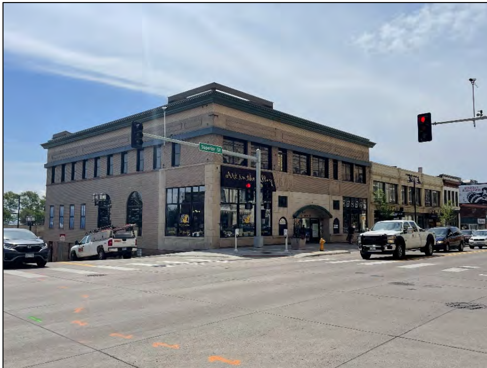
228-230 East Superior Street (Historic Name: Jacob Kohn Autos and Television Center Building)
