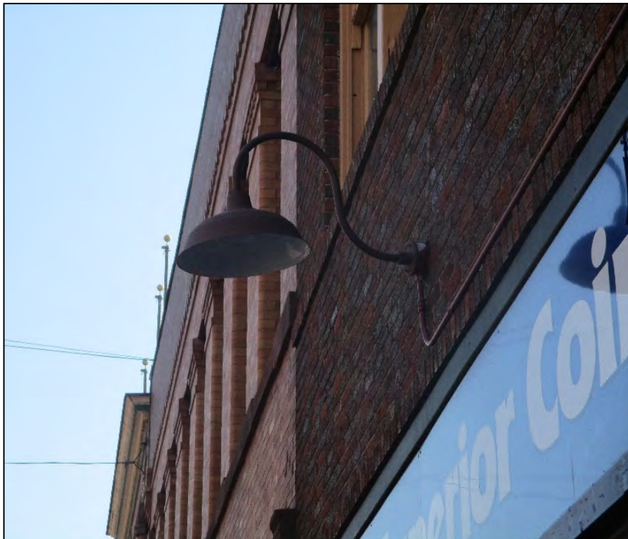
Photograph 21: View of historic gooseneck style lamp in the Duluth Commercial Historic District. Historic lighting should be maintained or replaced with updated light fixtures that replicate the originals.
