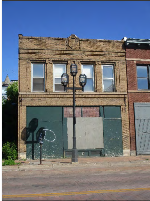
25 East 1st Street (Historic Name: Sher Bros. and Company)
