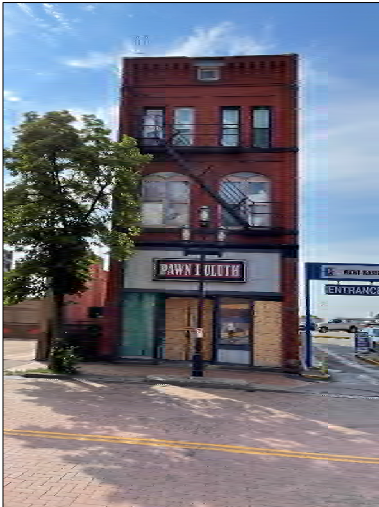
Photograph 22: View of 126 E. 1 st Street New stairways and fire escapes should not be added to the façade of historic structures within the historic district.
