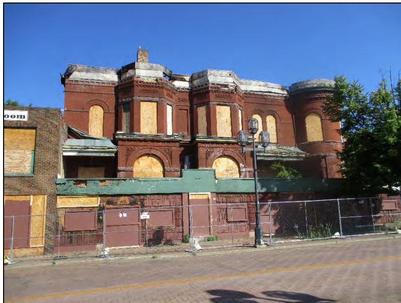
127-129 East 1st Street (Historic Name: Pastoret Terrace)
