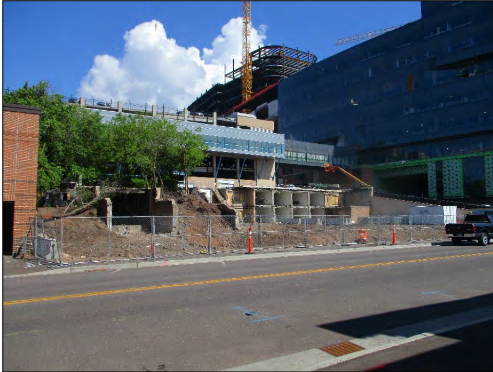
319-323 East Superior Street (Non-historic infill)
