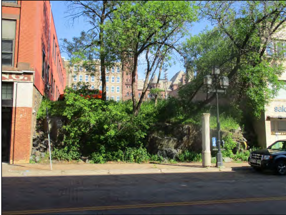
9 East 1st Street (Empty Lot with original granite retaining wall)
