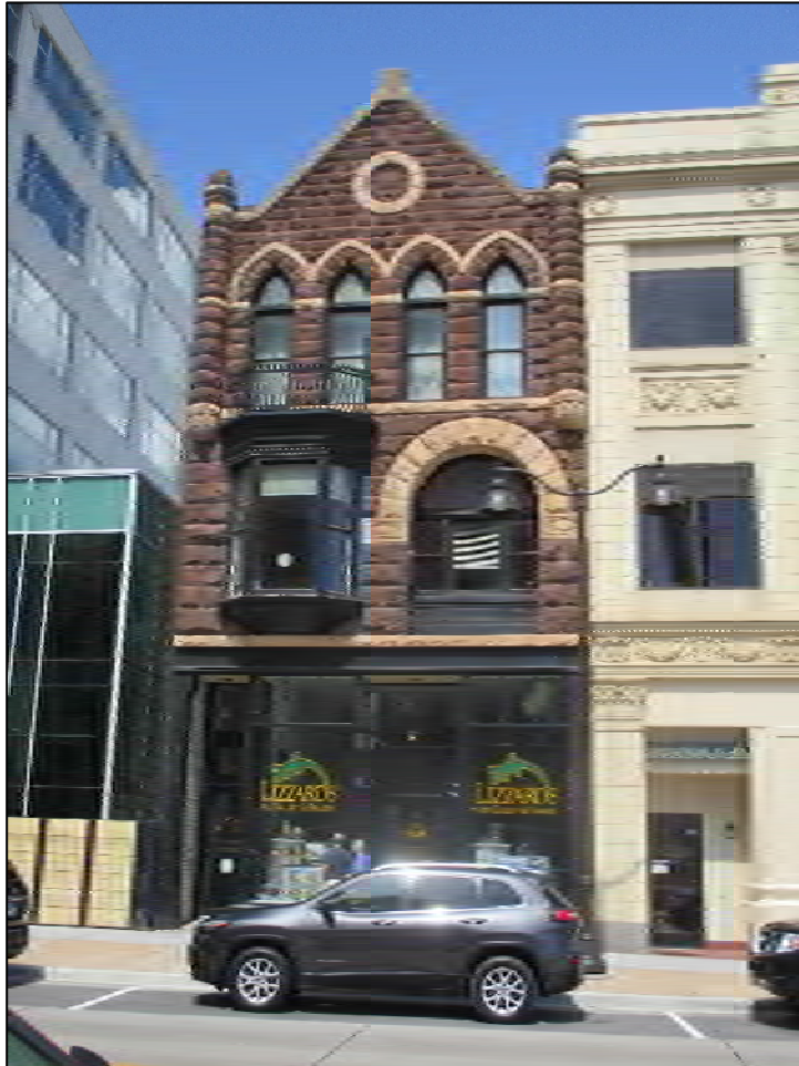
Photograph 6: View of the Gothic Revival building at 13 W. Superior Street. Note the gabled parapet and pointed arch windows at the third story.
