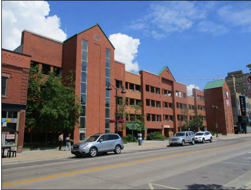
107-123 East Superior Street (Non-Historic Parking Structure)
