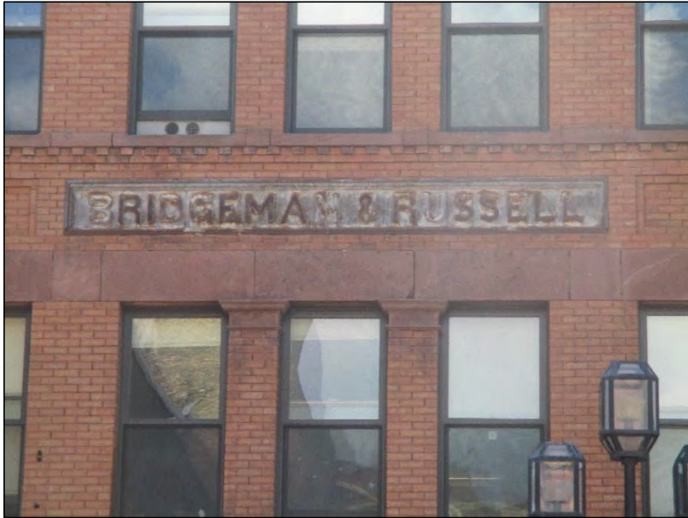
Photograph 29: Wall signs should be mounted above the storefront or on the façade between the storefront and cornice, like in the example here.
