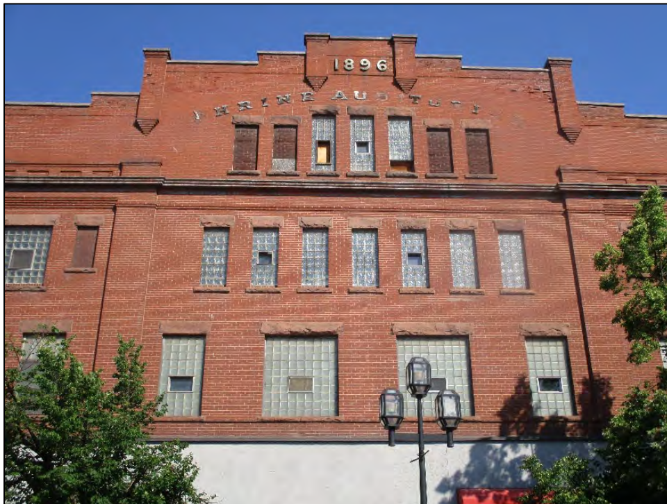
Photograph 12: Historic parapets such as the one seen on the historic Duluth Armory, located at 201-207 East 1 st Street, should be maintained.
