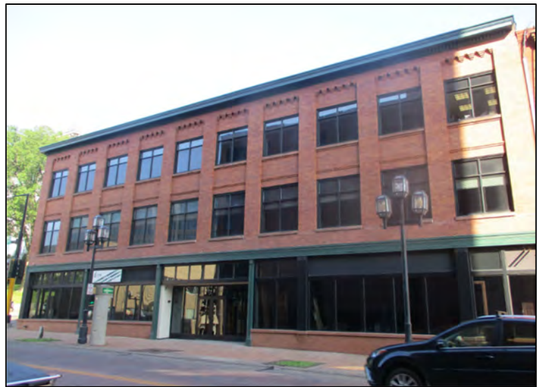
Photograph 3: View of the commercial building at 325 W. 1 st Street.
