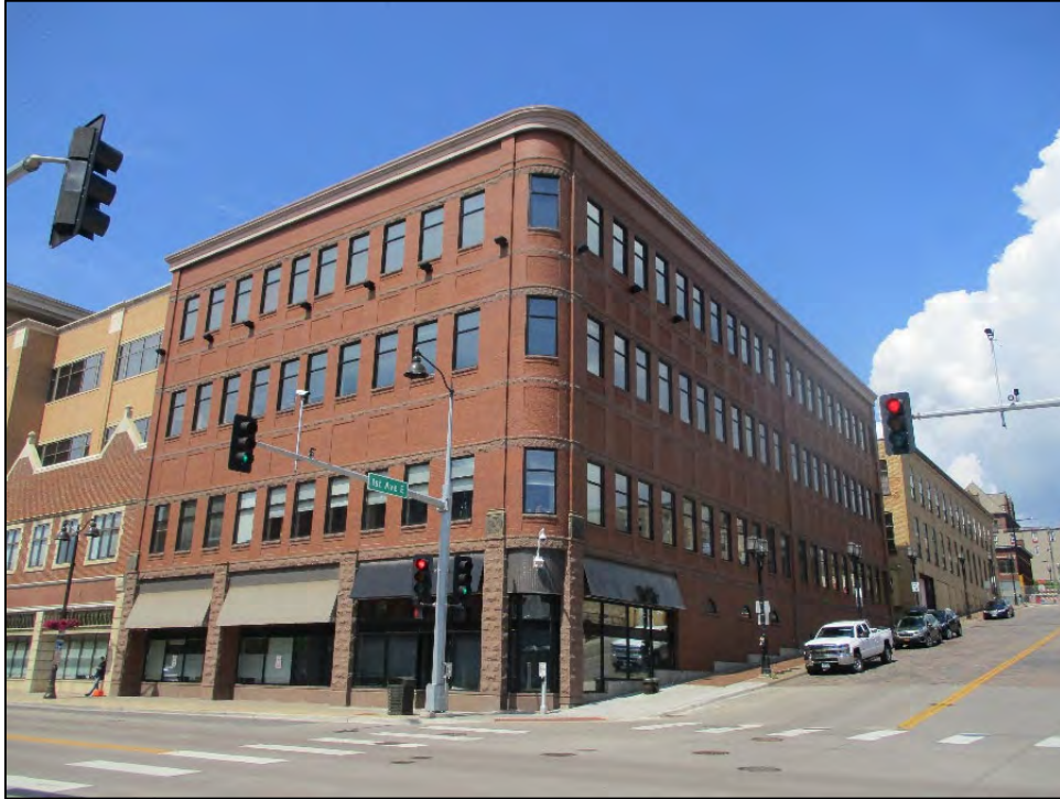
13 East Superior Street (Non-historic infill)
