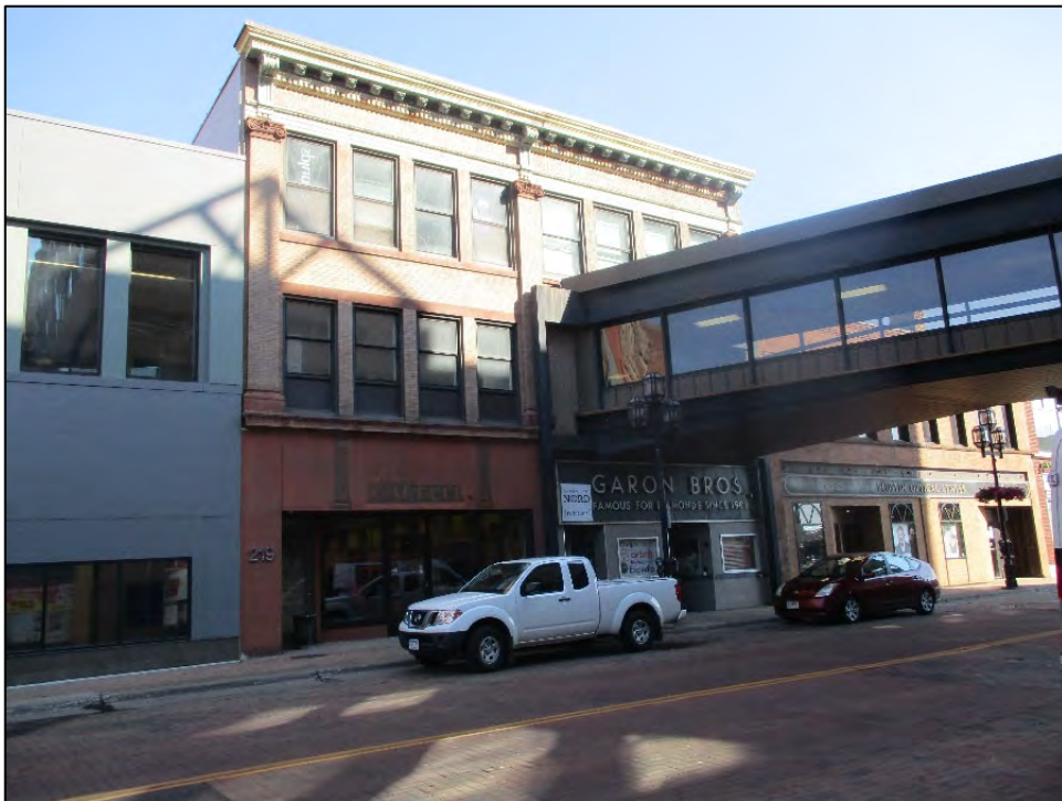
217 West 1st Street (Historic Name: Armstead Building)
