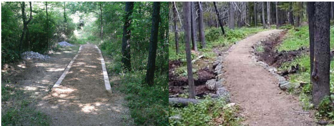
Figure 14: Causeway or Turnpike Trail Construction
