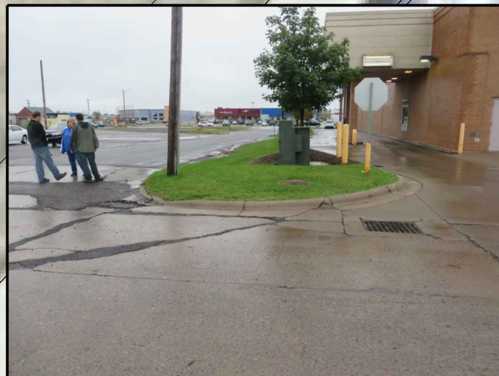
SITE OVERVIEW [LOOKING SOUTHEAST]
