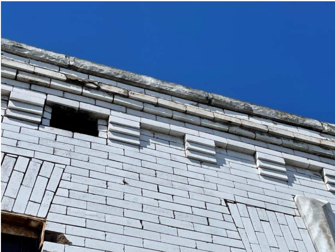
Photo 30: The existing parapets are deteriorated, missing or loose brick and exterior needs tuckpointing to prevent further deterioration.
