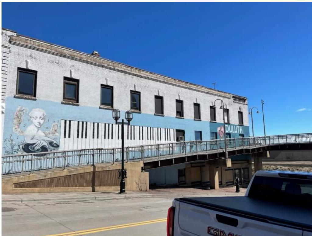
Photo 2: Existing West Elevation looking east
