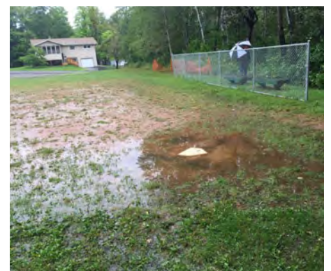
The existing ballfield has poor drainage
