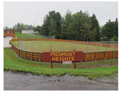
The lower rink is in new condition
