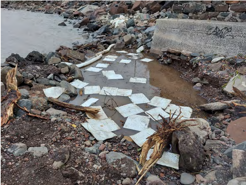
Initial area of impacted soils with booms and pads deployed, looking west.
