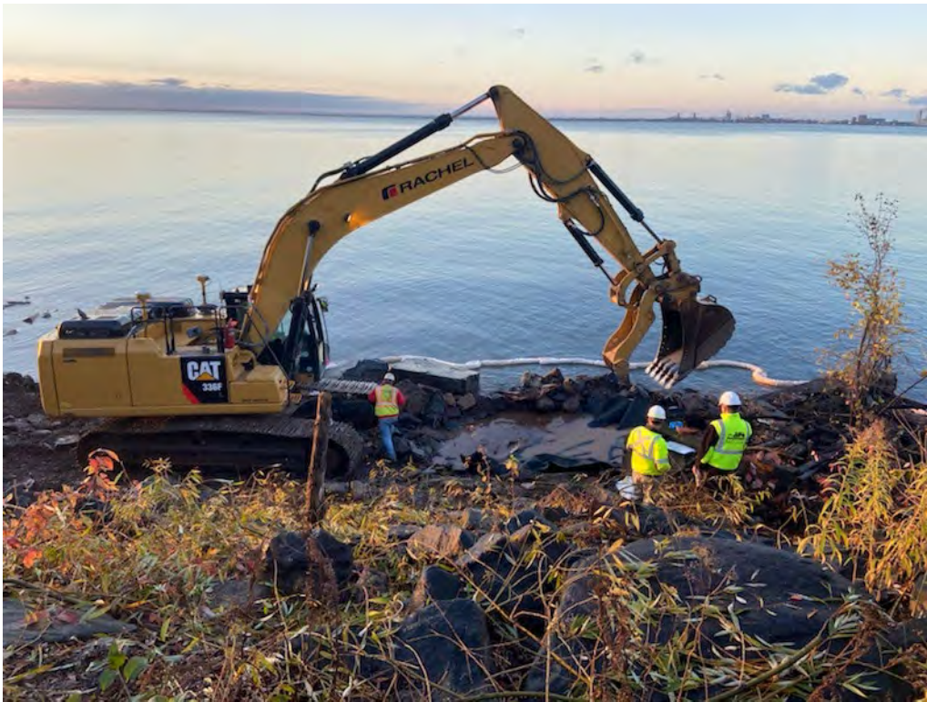
Excavation activity progressing to east along shoreline, looking south.
