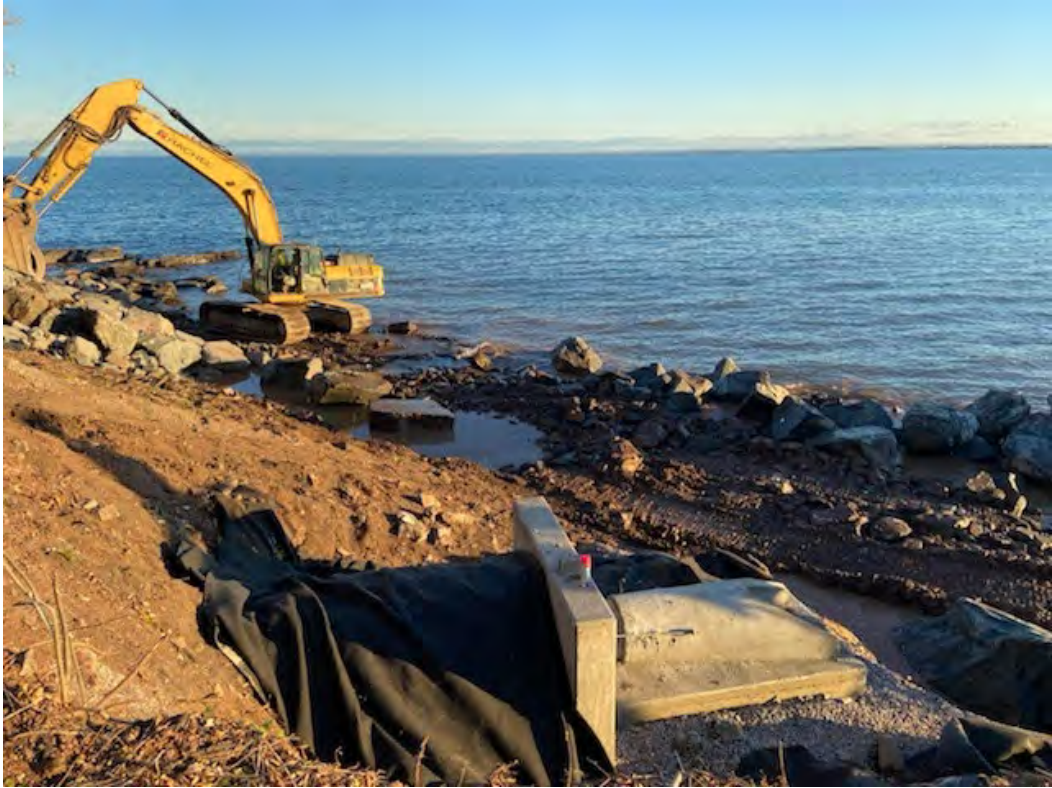
Backfilling excavation with shoreland armor foundation boulders
