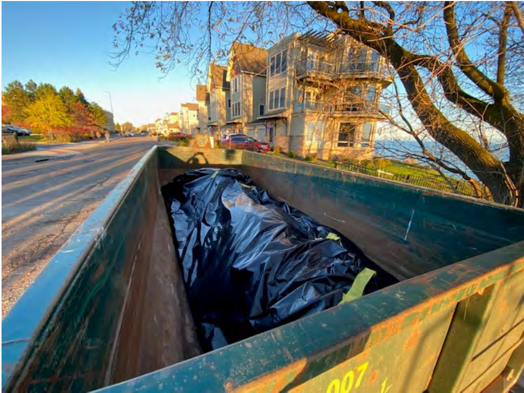
Impacted soils containerized in roll-off.
