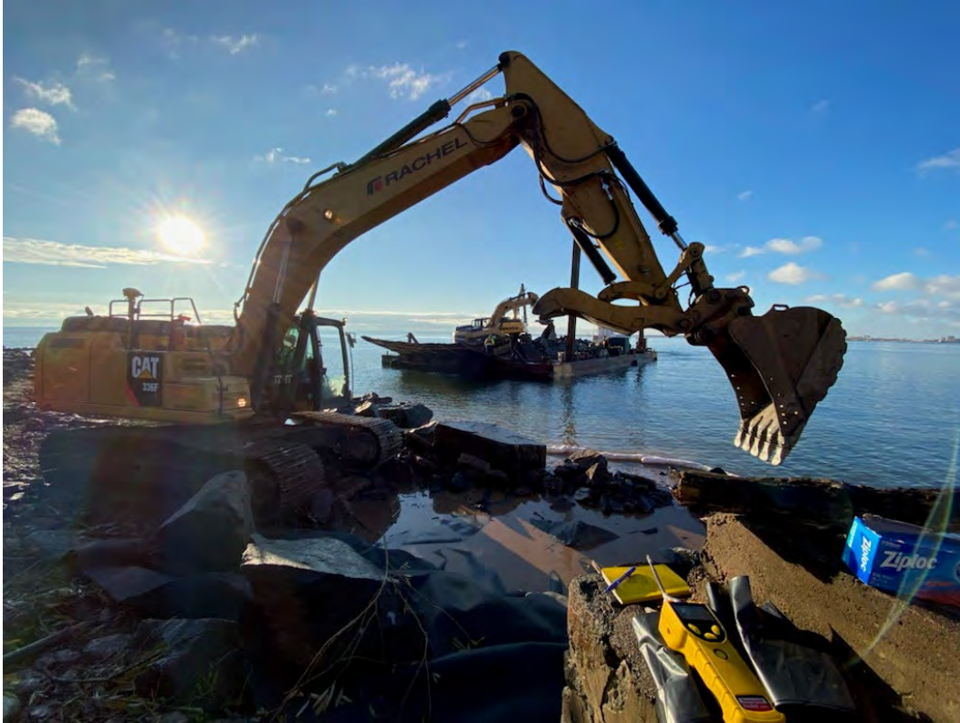
Excavation activity, looking southeast.
