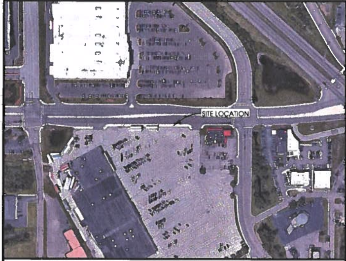
A AERIAL OVERVIEW
