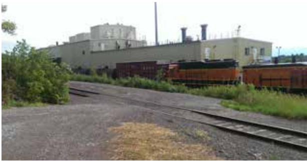
Figure 1.12 Existing Trail Crossing at Tate & Lyle site
