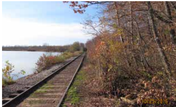
Figure 1.16 Segment 3 Existing Conditions
