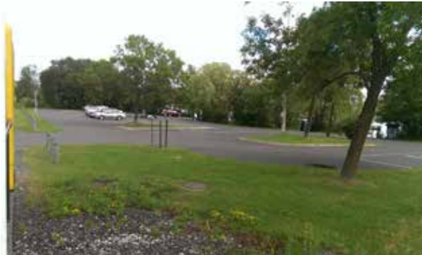
Figure 1.15 Segment 2 Existing Conditions
