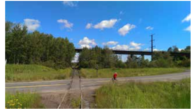
Figure 1.18 Segment 5 Existing Conditions
