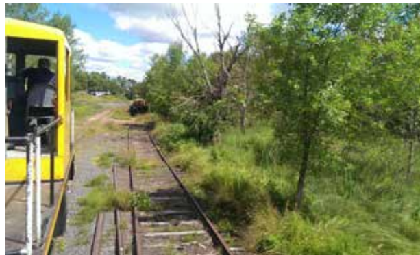
Figure 1.13 Segment 1 Existing Conditions
