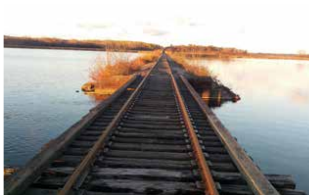
Figure 1.17 Segment 4 Existing Conditions
