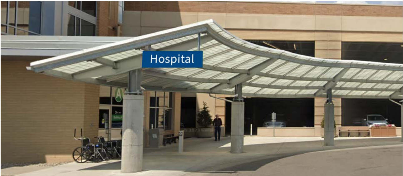
Hospital Entrance Canopy Reface existing hanging sign with new paint and vinyl graphics. Panel is painted Asprios brand blue, P1 . White vinyl graphics are matte white opaque vinyl applied to sign face - V2 . Provide field measurements of existing sign. KO&CO will provide final artwork in Adobe Illustrator format.
