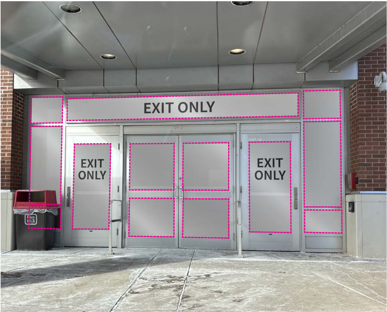
Old Hospital Building EXIT Dashed outlined areas above to recieve new printed and cut vinyl graphics and messaging on exterior. Translucent white vinyl applied to exterior of glass - VT3 . Cut matte black opaque vinyl applied over translucent white - V1 . Printed Aspirus leaf logo on opaque vinyl also applied over translucent blue vinyl. Replace 'Drop Off Zone' signs with new. Provide field measurements of all entrance glass as required for final layout of graphics. KO&CO will provide final artwork in Adobe Illustrator format.
