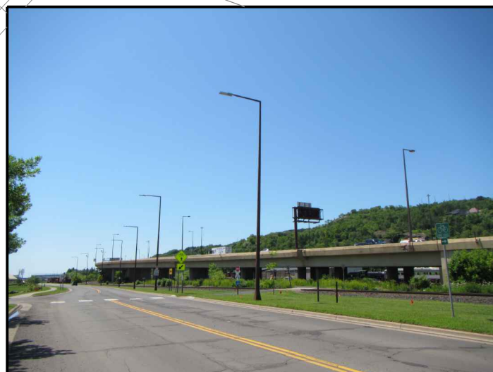
C SITE OVERVIEW [LOOKING SOUTHWEST]
