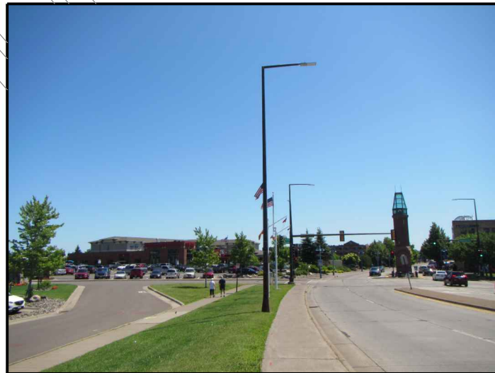
B SITE OVERVIEW [LOOKING SOUTHEAST]
