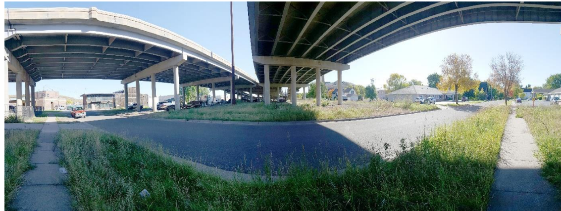
58 th Avenue Underpass below Interstate 35
