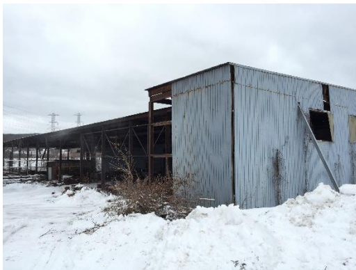
MN Steel Fabricators Site (Catalyst Site #4)
