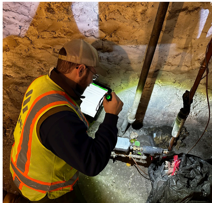
Documentation of a residence with lead service.
