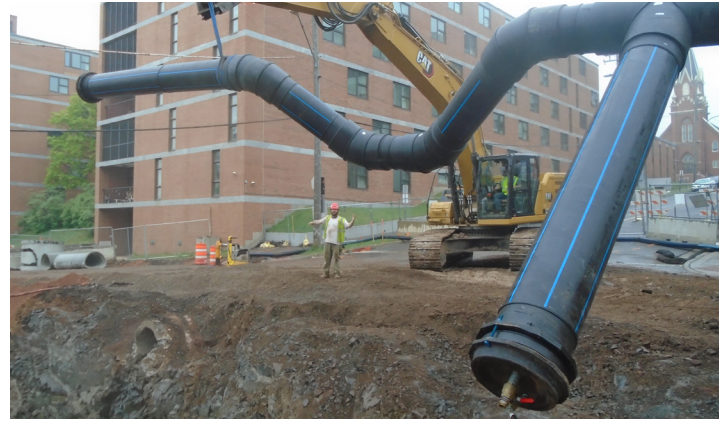
WEST MEDICAL DISTRICT INFRASTRUCTURE Essentia Health/City of Duluth/Mn Power | Duluth, MN
