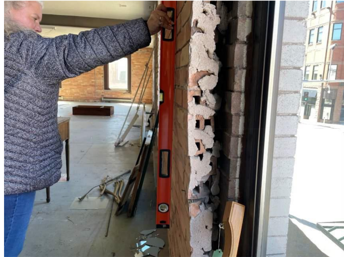
Photo 24: Existing north wall is bowed inward due to poor construction methods and water infiltration.
