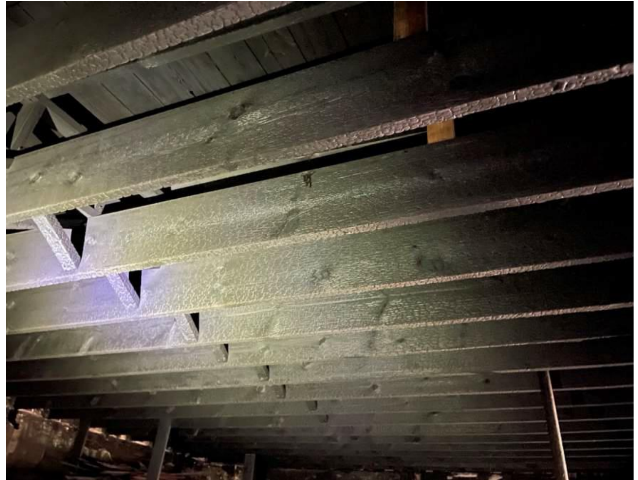
Photo 21: Existing roof joists that have been severely damaged due to fire.
