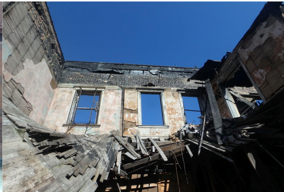
View from the inside of the 118 East 1 st St Street building looking towards 1 st Street. Note roof absence and second floor separation.
