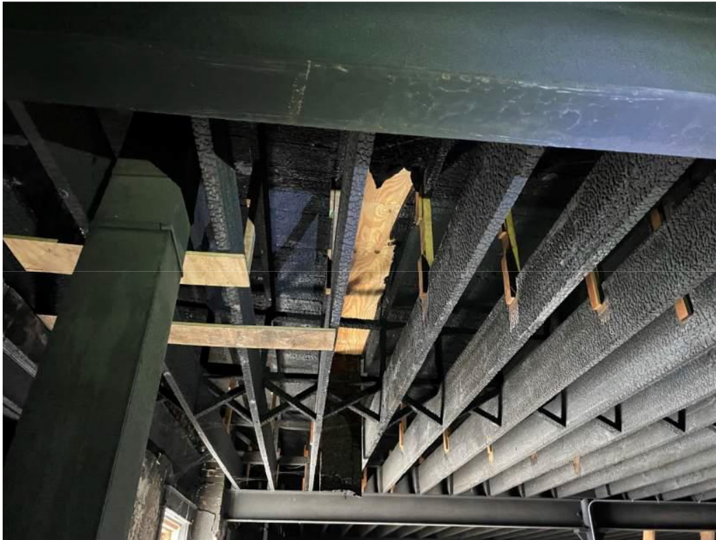
Photo 22: Existing roof joist framing severely damaged due to fire.
