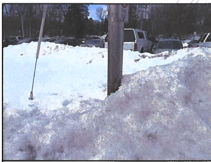
(C) POLE BASE [LOOKING NORTH]
