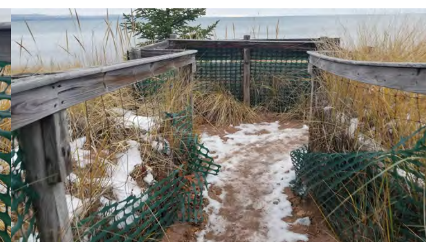
REMOVE FENCING AND WALL
