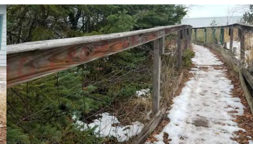
REMOVE FENCING AND WALL
