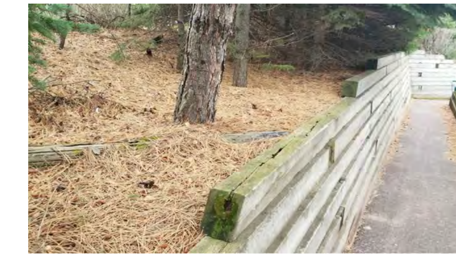
WALLS ON APPROACH RAMP - REMIAN
