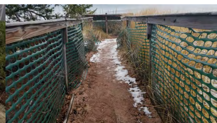
REMOVE FENCING AND WALL
