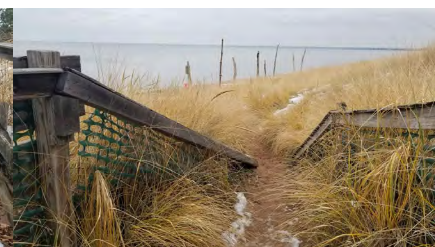
REMOVE FENCING AND RAILS
