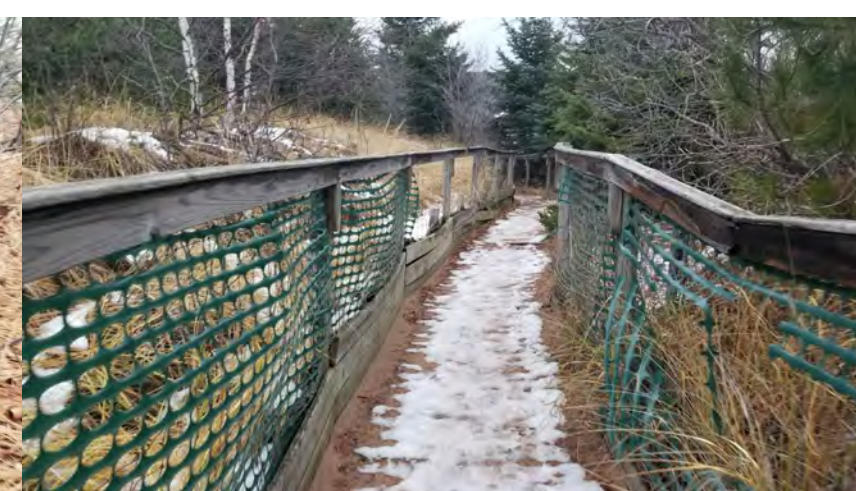
REMOVE FENCING AND WALLS BEHIND
