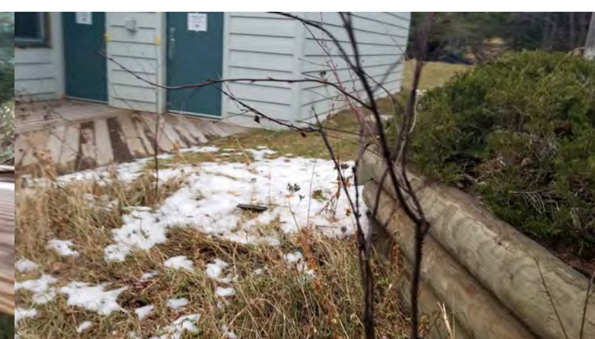
REMOVE FENCING AND WALL
