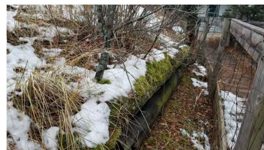
REMOVE FENCING AND WALL
