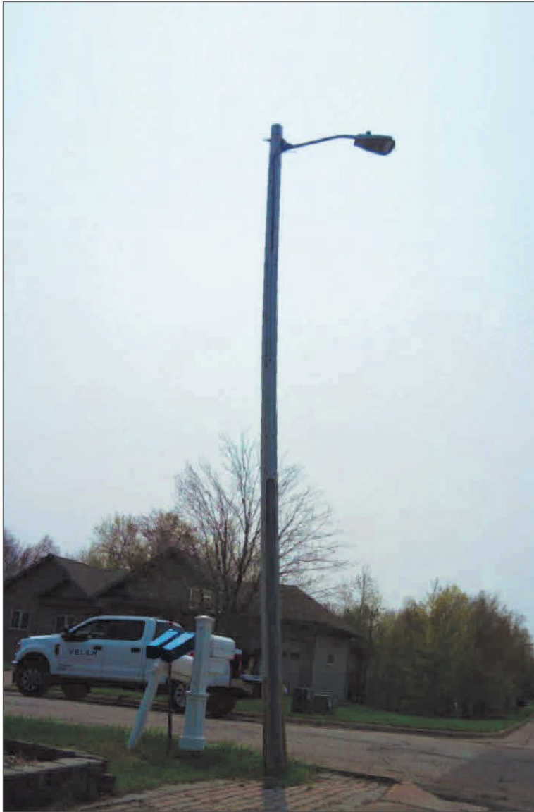
EXISTING SOUTH VIEW
