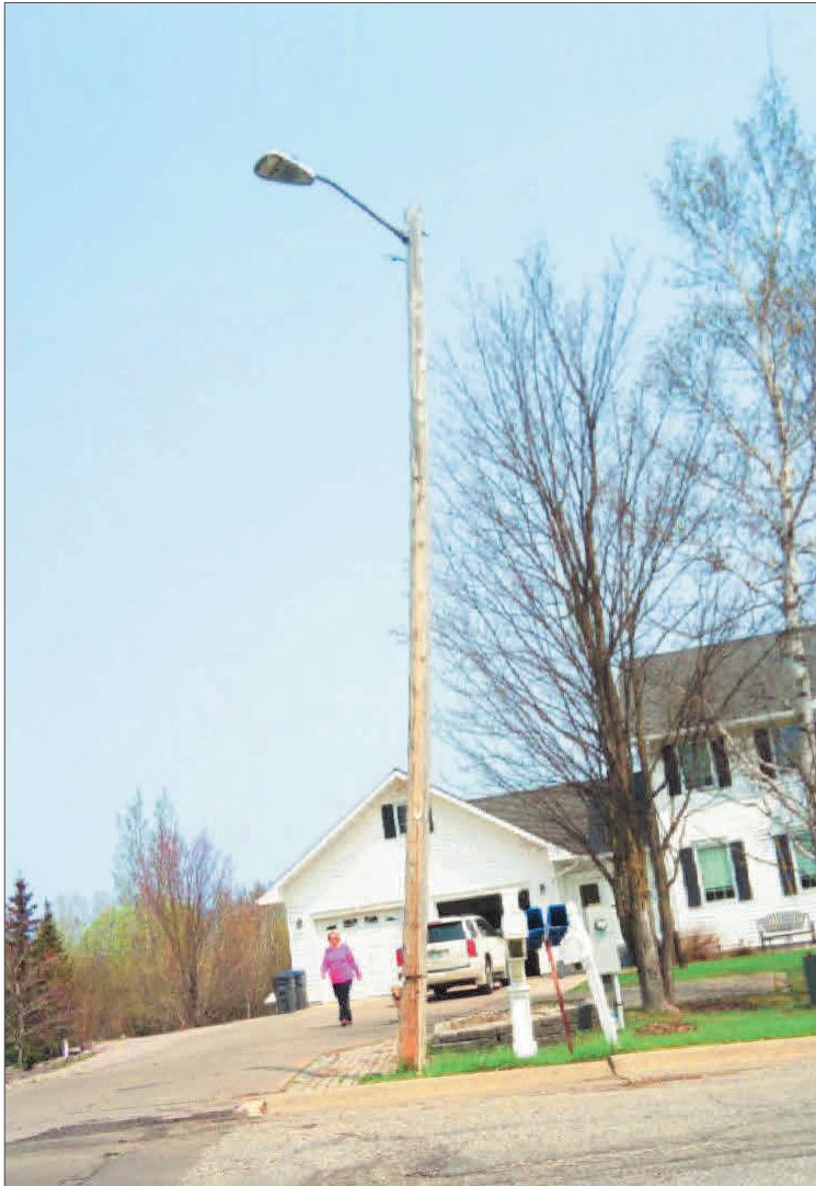
EXISTING NORTH VIEW
