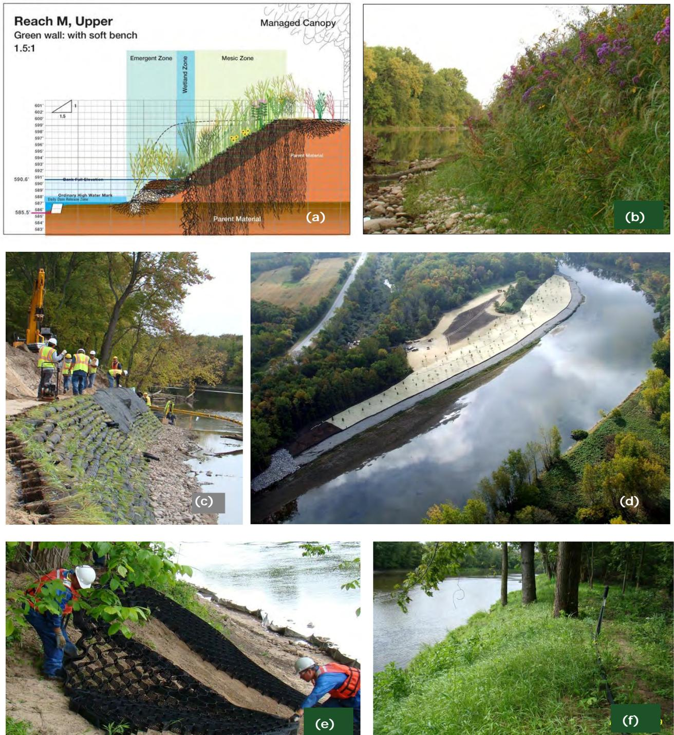
**Figure 3.** Bank stabilization measures in a Midwest river, subject to annual high-water flooding events. Examples include (a-c) use of geosynthetic bags and deep-rooted native plants (e.g., willows), (d) shoreline landscaping to include a hardened bank combined with constructed natural on-land habitat, and (e-f) geoweb-stabilized soils combined with deep-rooted native plants.
