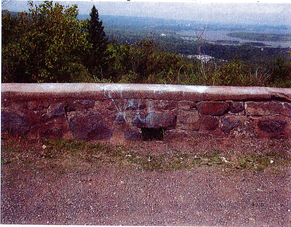
General parapet back face of wall— note drainage scupper
