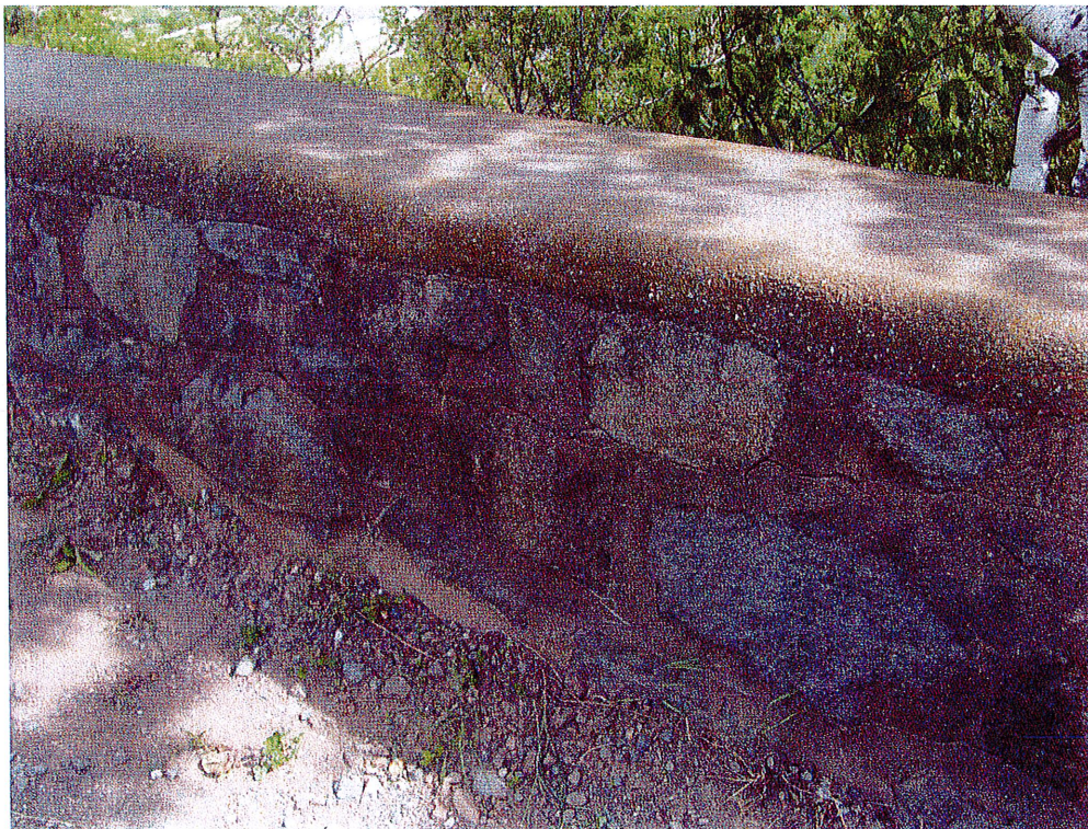
Poured concrete cap
