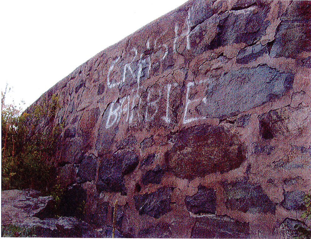
Front face of retaining wall – note separated mortar joints
