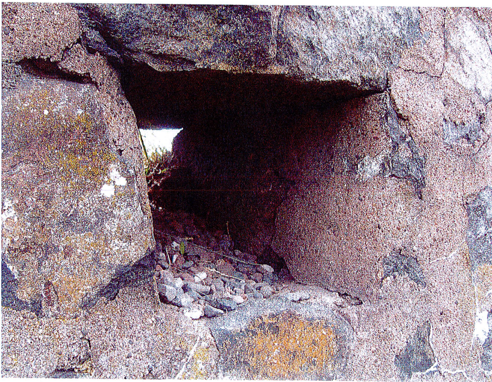
Drainage scupper, front face of wall
