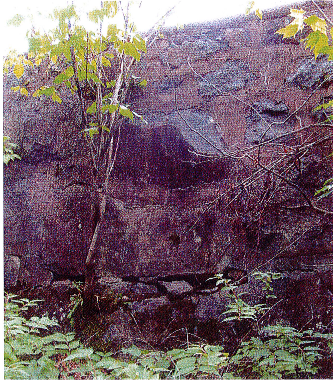
Front face of wall – note failed mortar joints with vegetation growth
