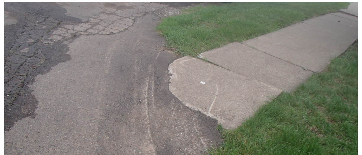
Pedestrian ramps will be reconstructed to provide better pedestrian access.
