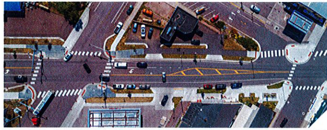
TH 61 GRAND MARAIS RECONSTRUCTION MnDOT | Grand Marais, MN
