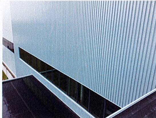
New wall panels have been installed
