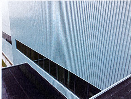
New wall panels have been installed
