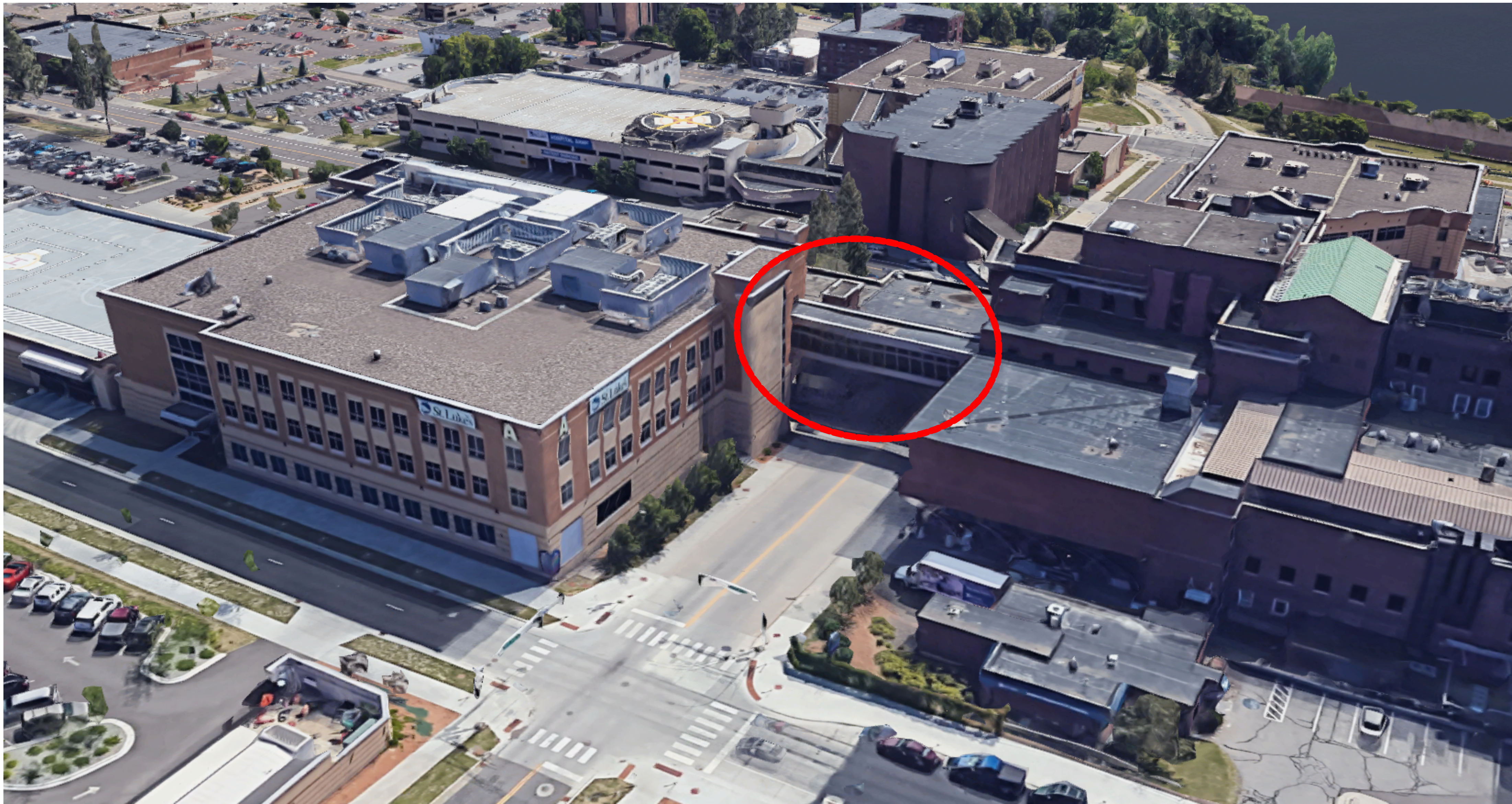
2 SITE CONTEXT - LOOKING EAST SCALE: 12" = 1'-0"
