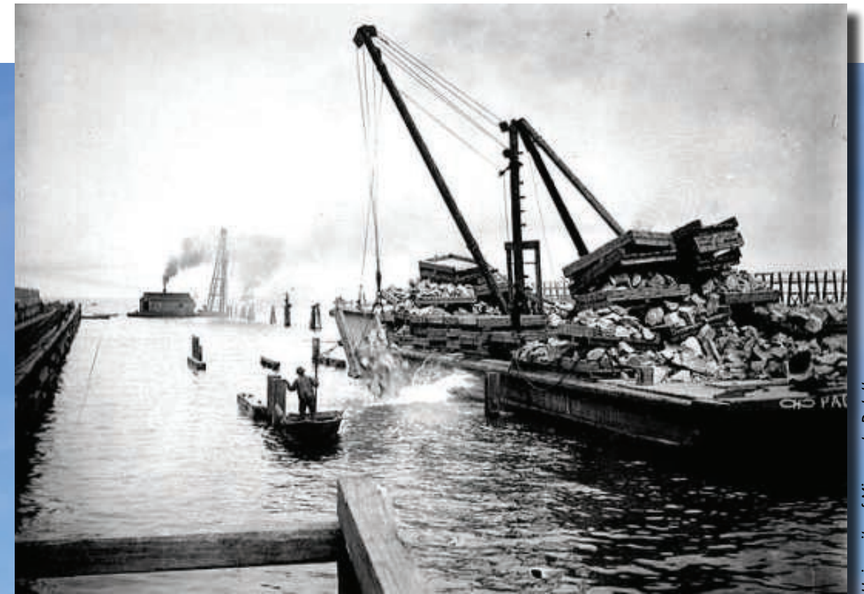
The Construction of the Shipping Canal, 1871
