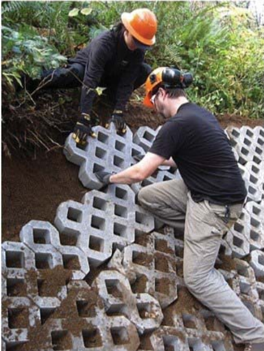
Figure 6: Turf Block Pavers
