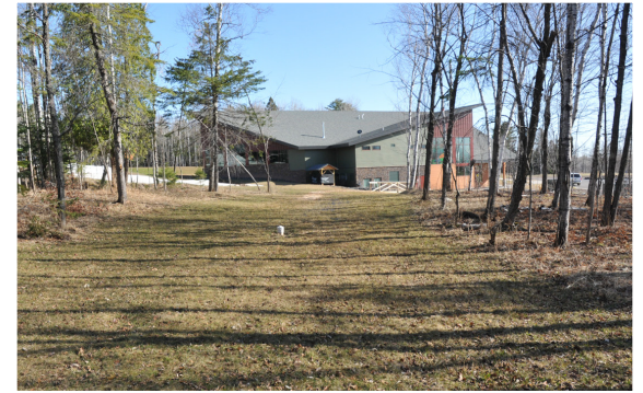
Chalet from staging area.
