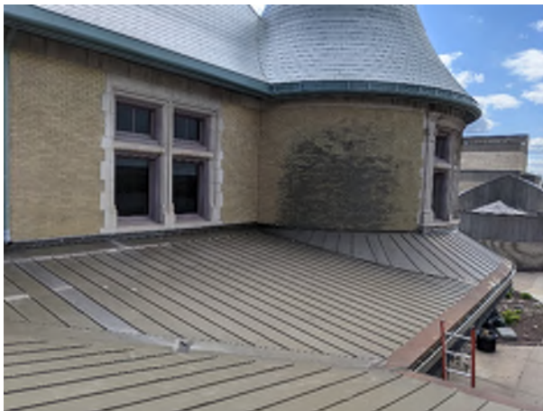
PICTURE #9 Roof Standing Seam
