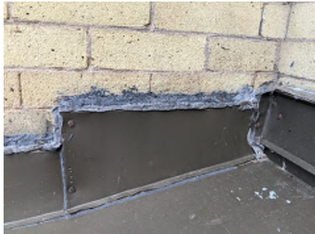
PICTURE #14 Roof/Wall Flashing
