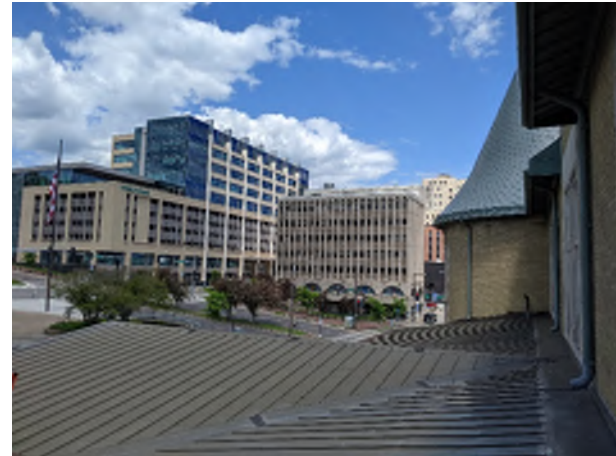
PICTURE #10 Roof Standing Seam
