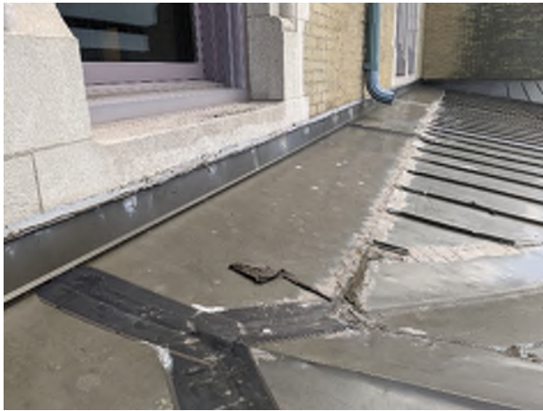
PICTURE #11 Roof/Sill Flashing
