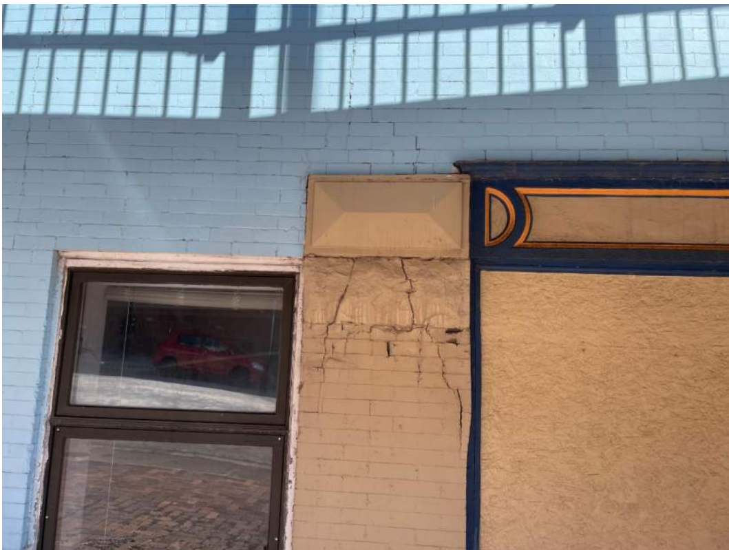
Photo 8: Close-up view of brick condition on west exterior wall looking east
