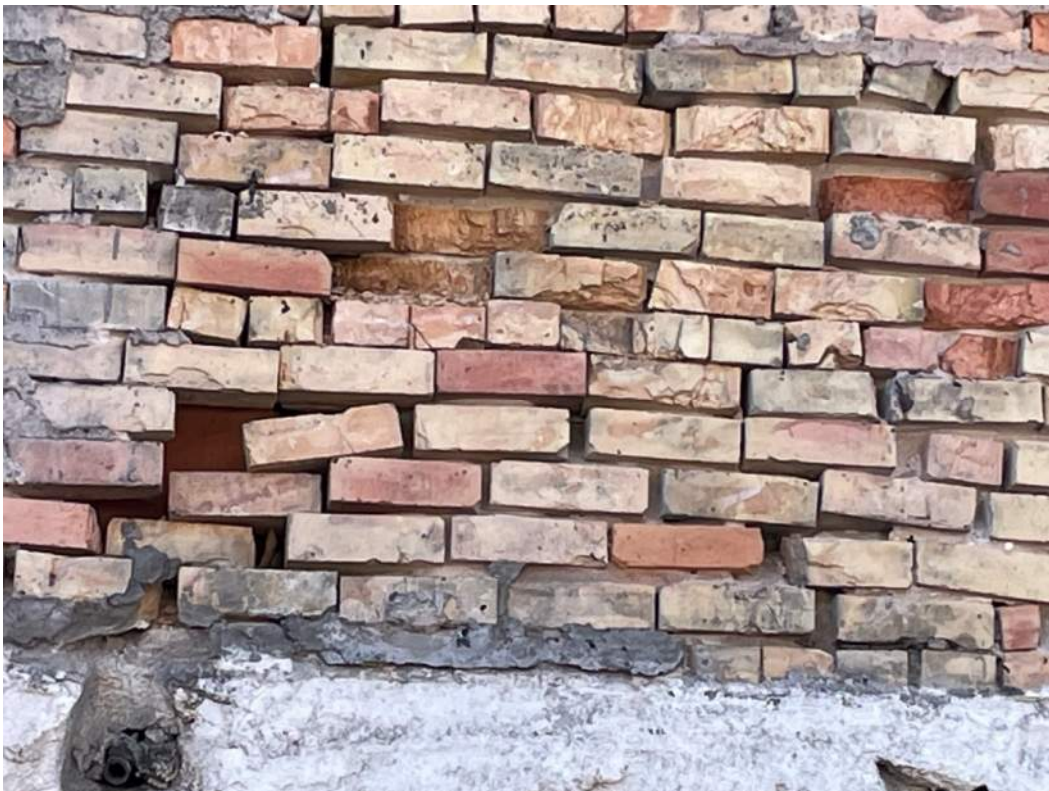
Photo 12: Close-up view of existing east exterior wall masonry condition
