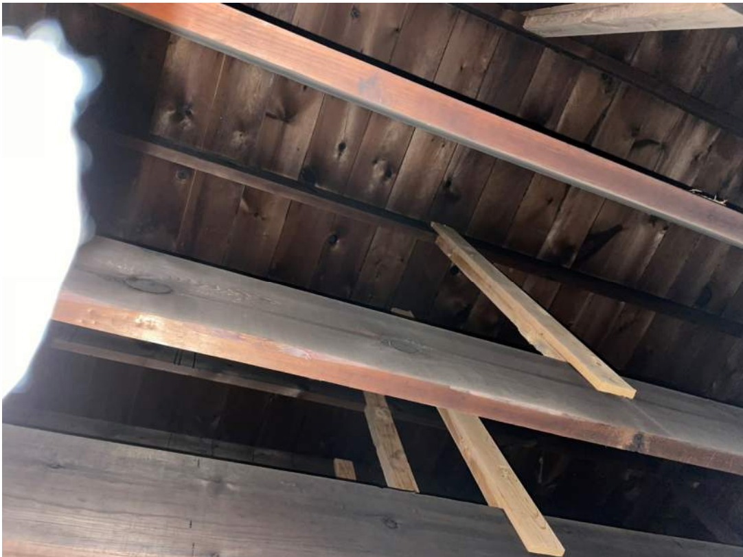
Photo 20: Existing ceiling joist and roof joist system does not meet current code for snow load, is currently not insulated.
