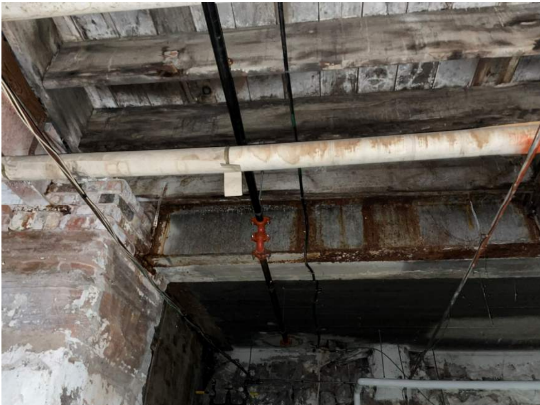
Photo 14: Existing sidewalk vault support and existing wood floor framing near entrances is generally in poor condition
