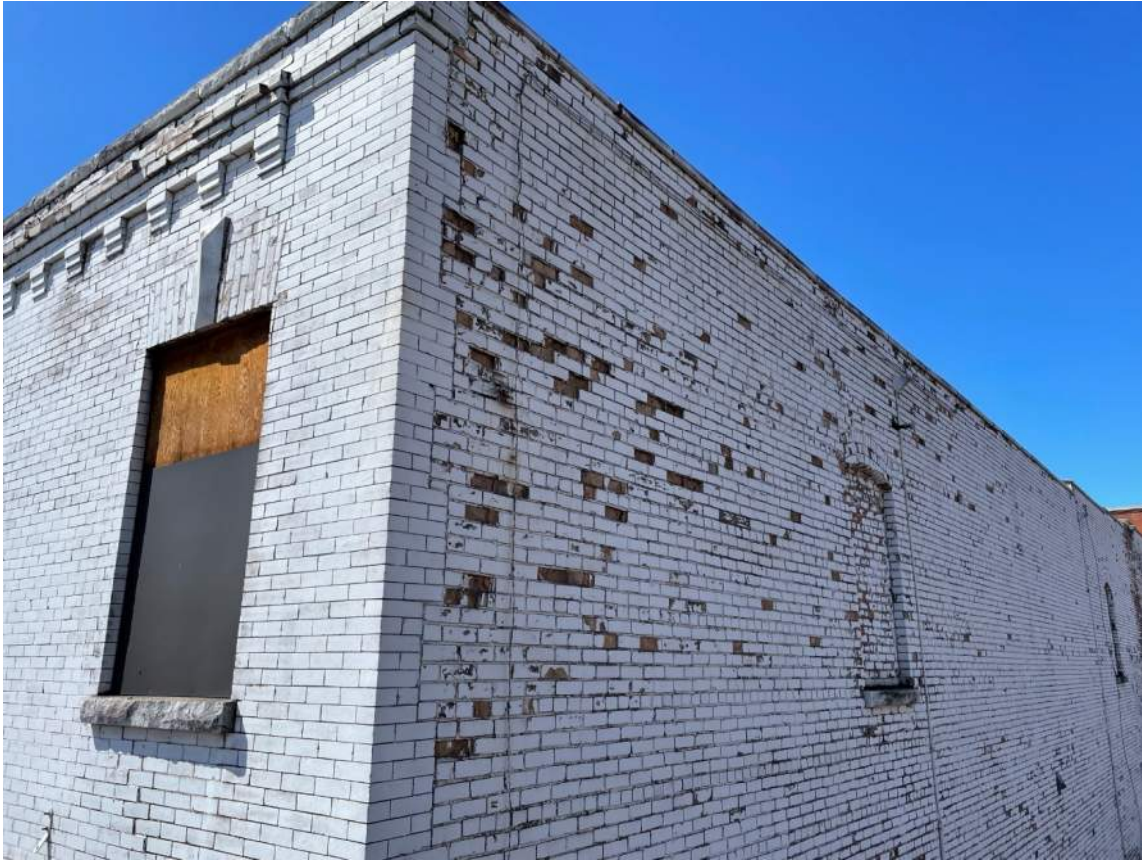
Photo 31: Exterior southeast corner – note the spalling brick due to moisture intrusion, freeze thaw cycles causes a spall, which falls to the ground.
