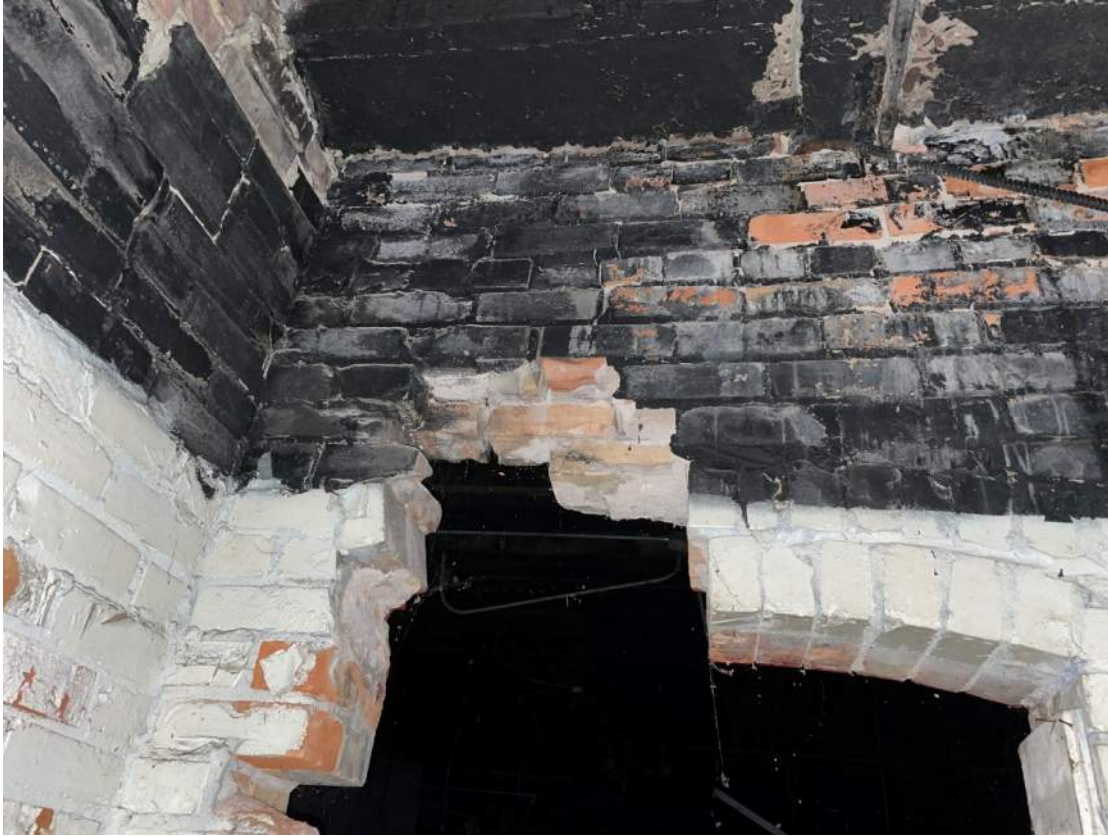
Photo 15: Existing sidewalk vault support is generally in poor condition
