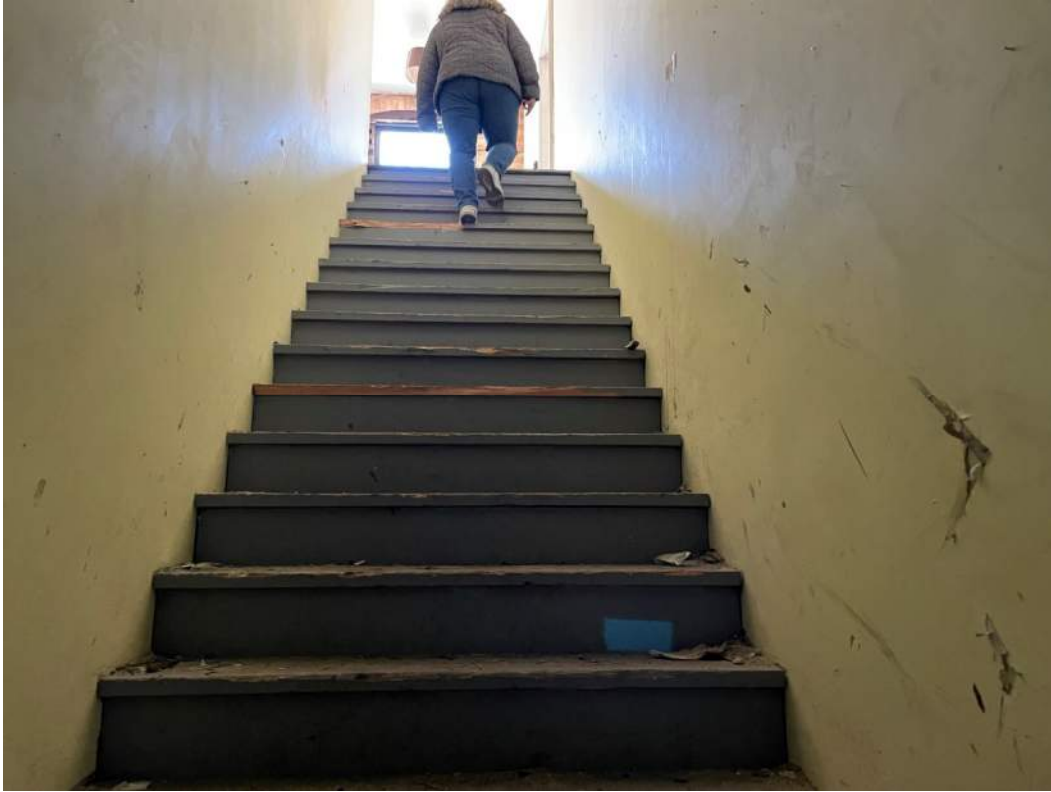
Photo 19: Interior stairs are not to current code rise / run or fire separation issues and would need to be replaced if major renovation were undertaken
