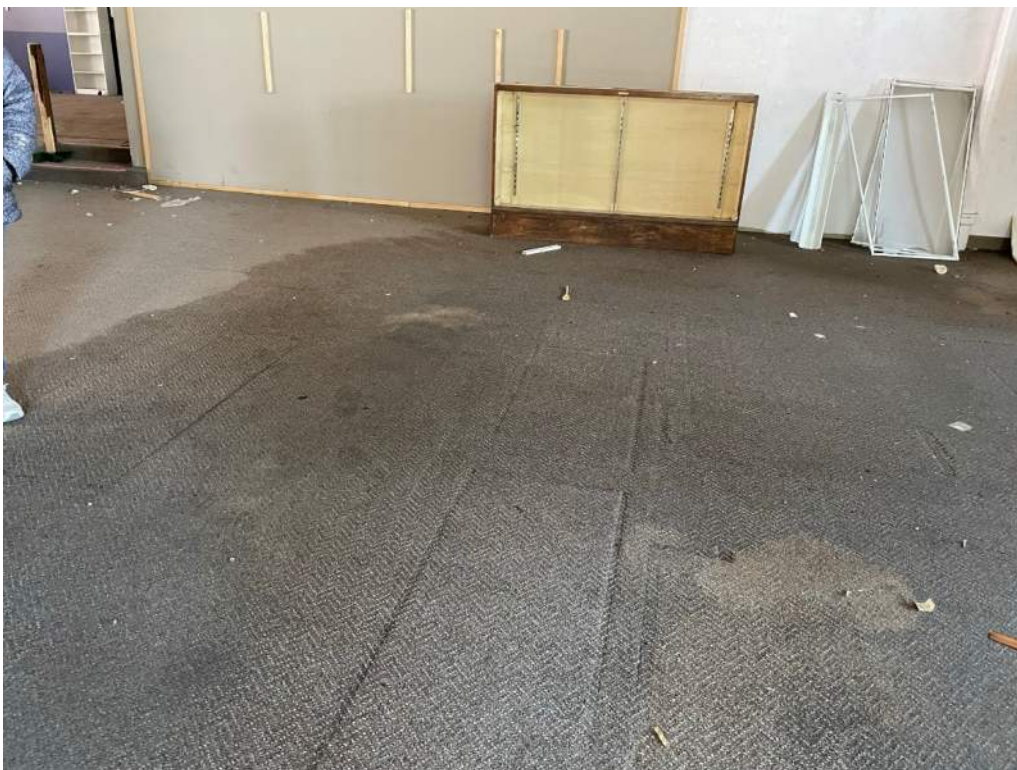
Photo 18: Rainwater on the upper floor level due to deteriorated roofing.
