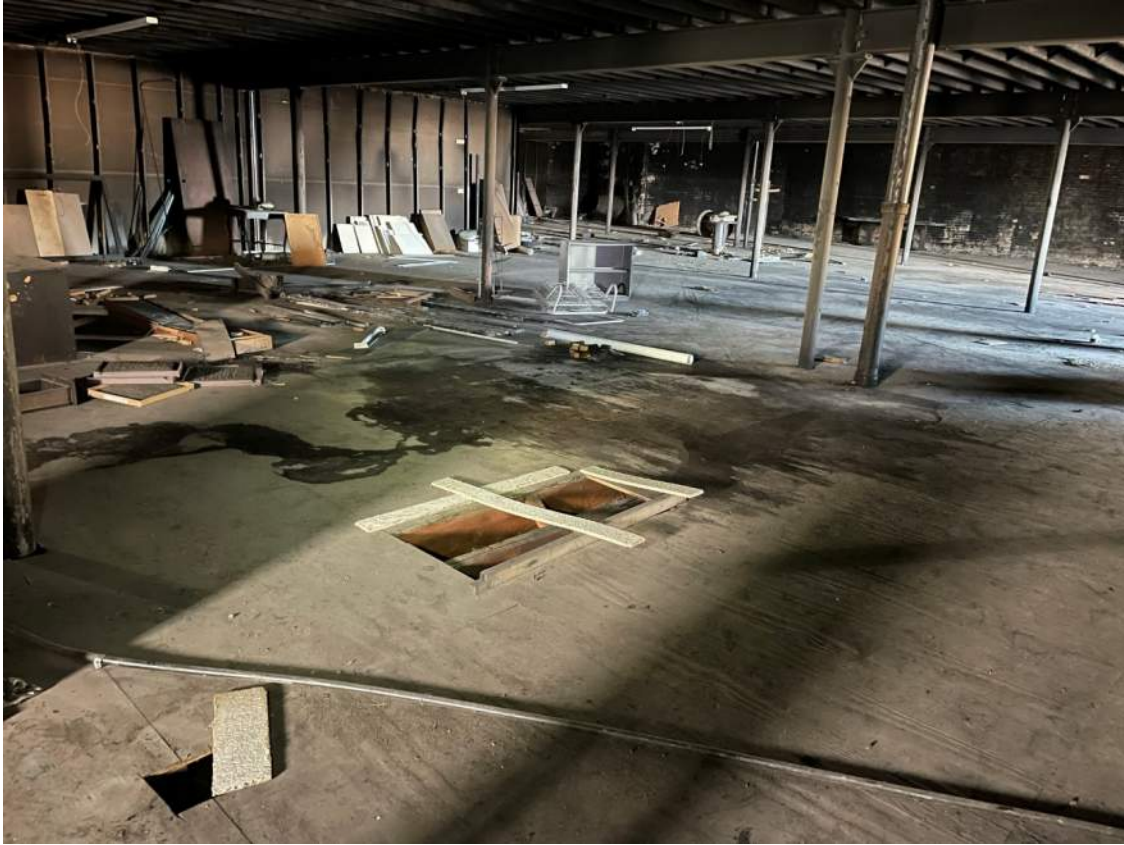
Photo 23: Existing wet flooring on the upper level due to roof leaks.
