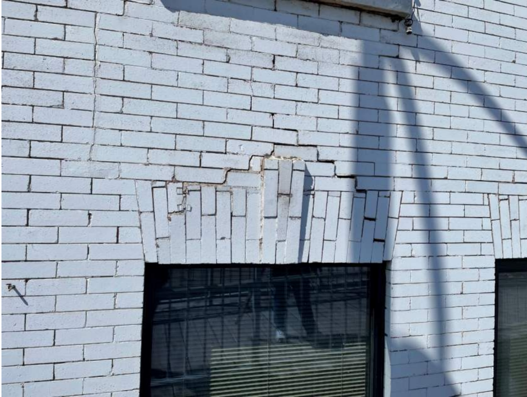
Photo 29: Typical exterior lintels are loose and failing and require replacement
