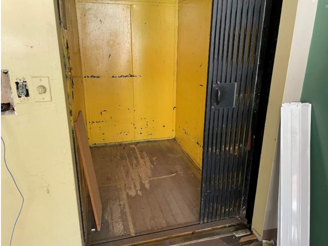
Photo 25: Existing freight elevator, would require significant upgrades or replacement if a significant renovation were to occur.
