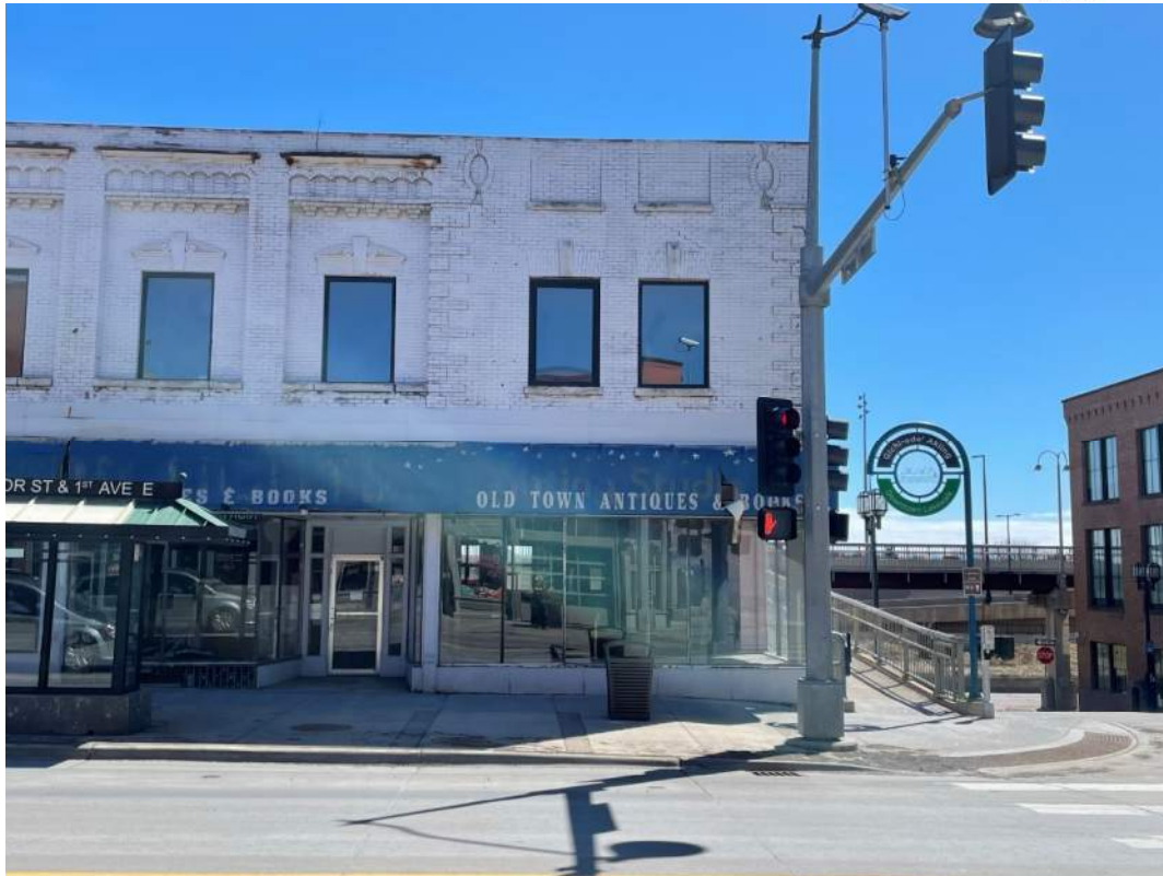
Photo 3: North exterior wall looking south
