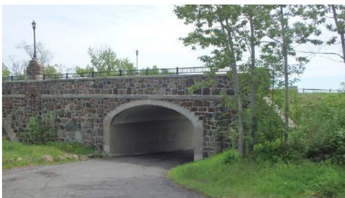
Poor approach sight lines for vehicular and pedestrian traffic at 10th Street bridge underpass
