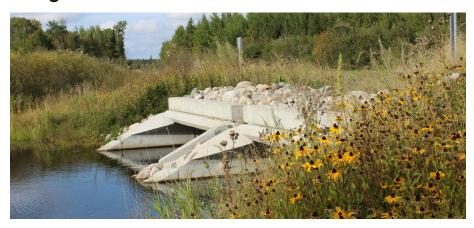
LHB provided preliminary and final design services for the replacement of St. Louis County Bridge No. 709, carrying County Road 769 over the Willow River south of Orr, MN. The old bridge, built in 1970, was a single steel beam span with timber plank deck and timber abutments. During annual safety inspections, it was observed that the timber abutment
