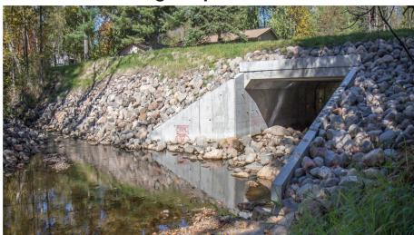
washed out the existing multiple pipeculvert type bridge carrying Toledo Street over Chester Creek in Duluth, MN. LHB was hired to perform a hydraulic study and preliminary and final design of the new structure. Based on hydraulic performance, durability and cost a precast concrete box culvert was chosen as the most appropriate structure for this
