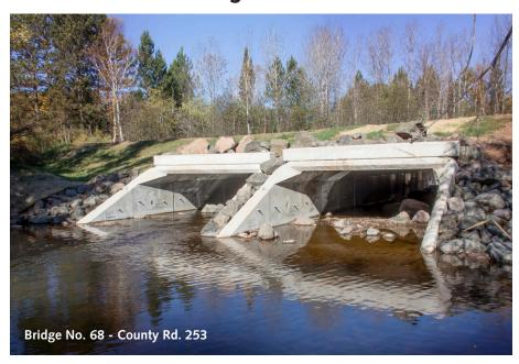
Following the June 2012 Flood, LHB was hired to coordinate design and construction for 15 flood damaged structures in Saint Louis County. Three of those structures (Bridges 67, 68 and 846) are located within a few miles of each other and all cross the Little Knife River. Based on site conditions, low traffic volume, and hydraulic demands, LHB
