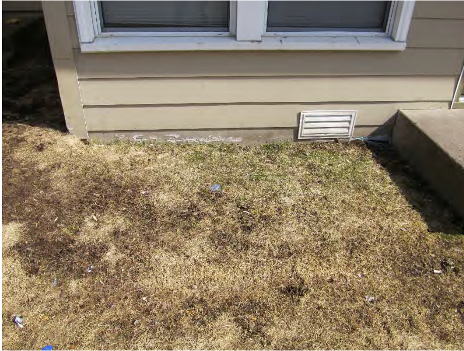
Figure 5 Fiber cement into the soil and at uphill location. Note typical deterioration of siding at this location
