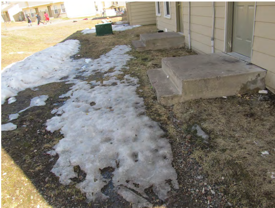
Figure 10 Stoop condition, solid but some grease stains
