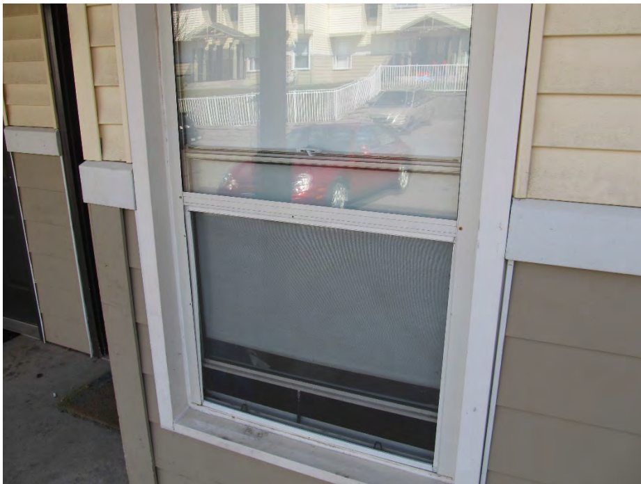
Figure 6 Oldest window type, one latch. Note pencil for support
