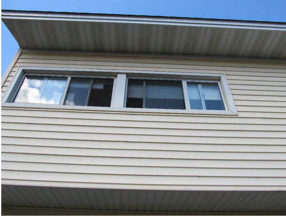
Figure 3 Soffit and trim in good condition as us upper siding of vinyl.
