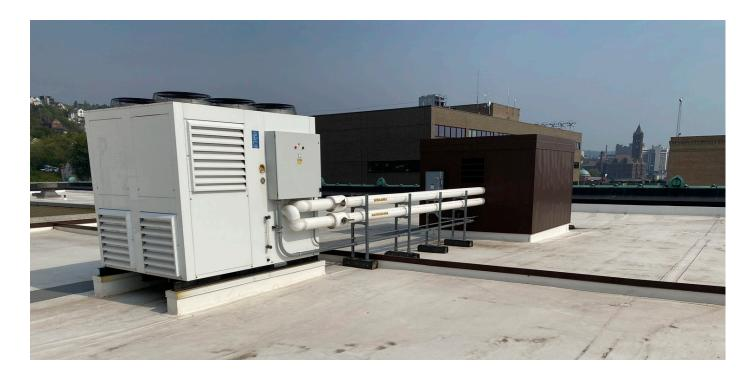
unit from structure improvements on the low roof to minimize required screening. KFI has worked with many manufacturers to minimize noise pollution caused by chillers. Specifying low sound fans, condenser blankets, and sound louvers, in addition to maintaining energy efficiency from the equipment.
