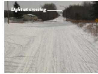
Along with proper signage, a light is added at this trail crossing to improve safety. The flatness and straightness of this trail conversion reduced the visual cues associated with identifying this intersection, warranting the addition of the light.
