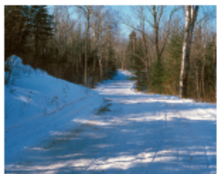
Longer, flowing curves with adequate sightlines are preferred for snowmobile trails. Sightlines should be long enough for the rider to react to oncoming conditions but not so long as to entice excessive speeds.
