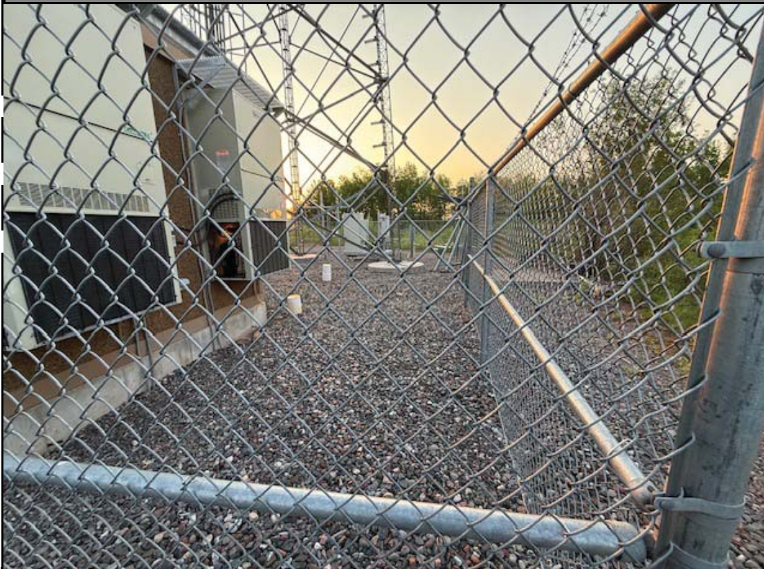
VIEW OF THE SITE FROM THE WEST
