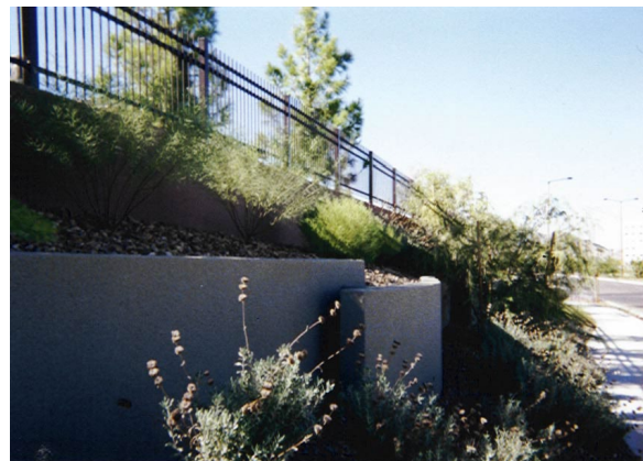
Figure 50-26.4-B: Retaining wall terracing and articulation
