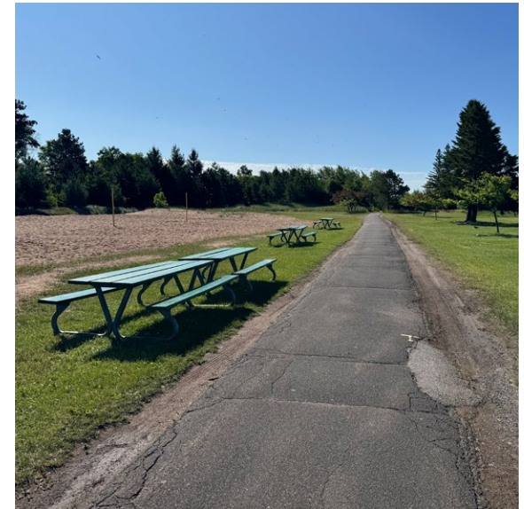
Figure 02.26 Existing path in front of sand volleyball courts
