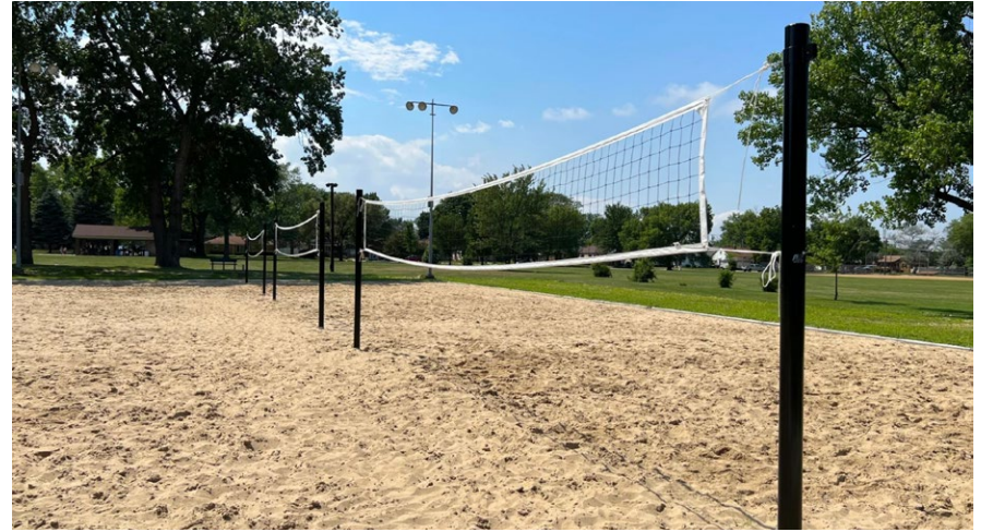
Figure 04.6 Natural sand volleyball court example with new posts, nets and edge perimeter
