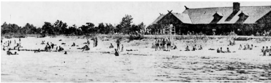
Figure 01.6 View of the bathhouse, 1939. "New Park Point Bath House Opens", June 24, 1939 Duluth News Tribune, newspapers.com
