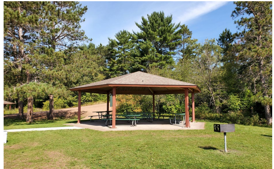
Figure 04.8 Current picnic shelter with amenities available for rental
