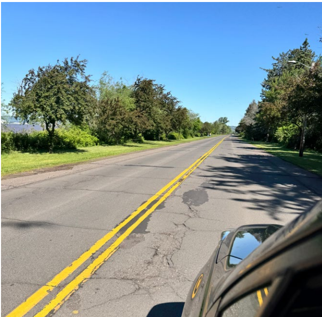
Figure 02.10 Existing road conditions at park entrance (left)
