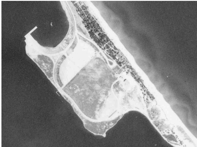
Figure 01.7 Aerial of the recreation area, September 12, 1940. Image credit: Minnesota Historical Aerial Photographs Online, John R. Borchert Map Library, University of Minnesota.
