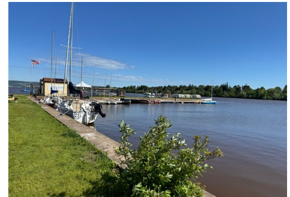
Figure 02.15 Sailing pier with seawall
