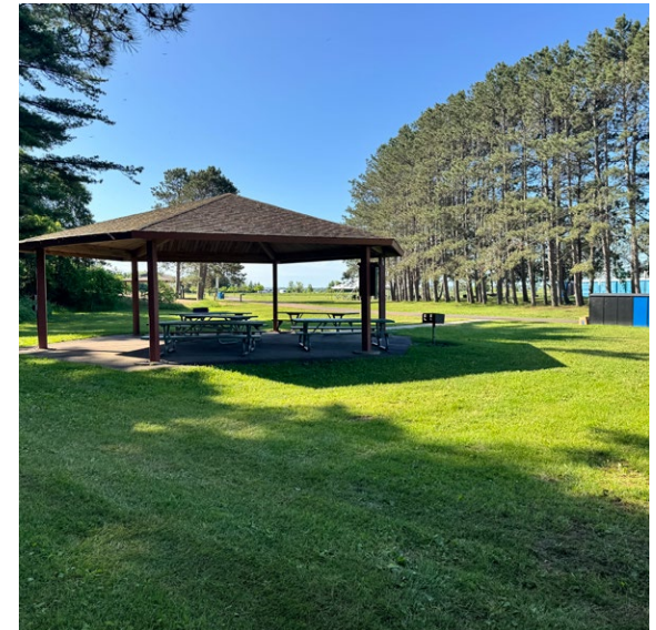
Figure 02.24 Existing picnic shelter
