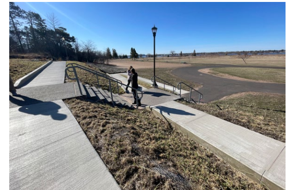
Figure 02.39 New accessible ramp at Beach House
