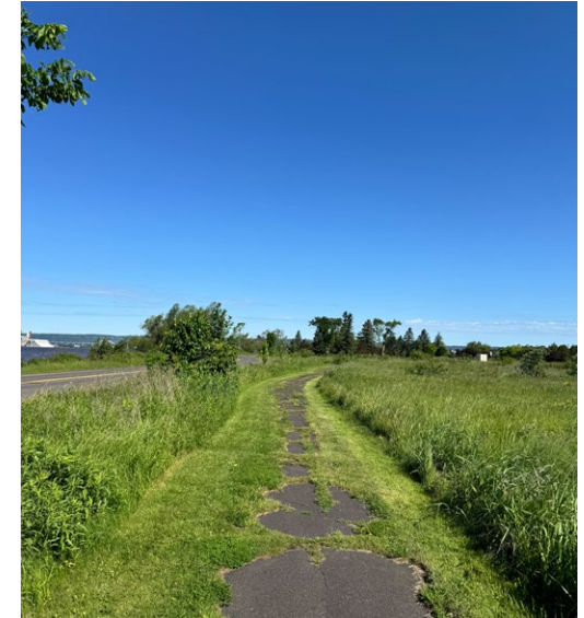
Figure 02.6 Paved pedestrian path
