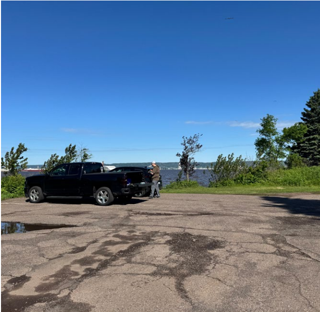
Figure 02.18 Trailer parking flooding (left)
