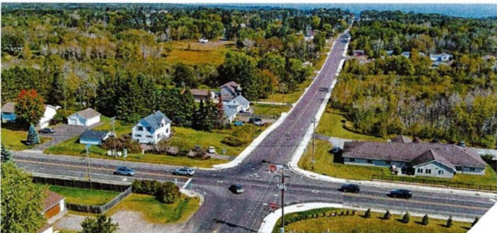
MORRIS THOMAS CSAH 56 BETWEEN HAINES & PIEDMONT RECONSTRUCTION St. Louis County | Duluth, MN
