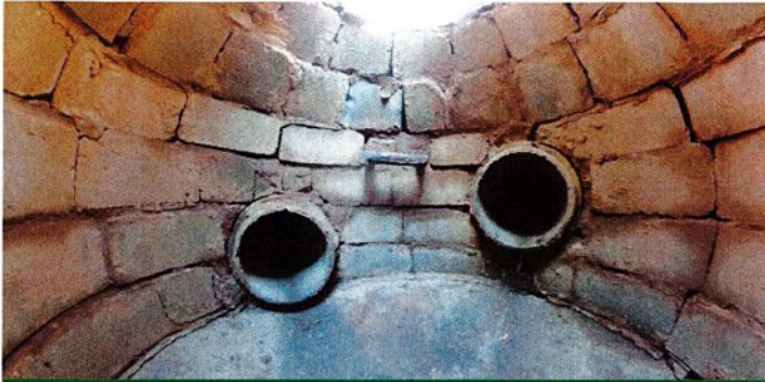
Example of 360-degree image taken during the City of Duluth's Morley Heights project.
