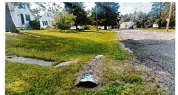
Existing heaving driveway culvert on Springvale Road.
