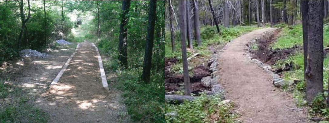
Figure 14: Causeway or Turnpike Trail Construction
